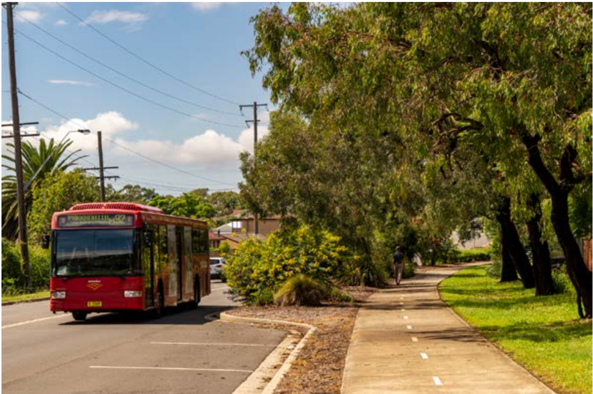
Menai Road was bypassed by Bangor Bypass. It was subsequently posted at 50km/h with a narrower road width and trees, vegetation, footpath and car parking bays included into the reclaimed space.
