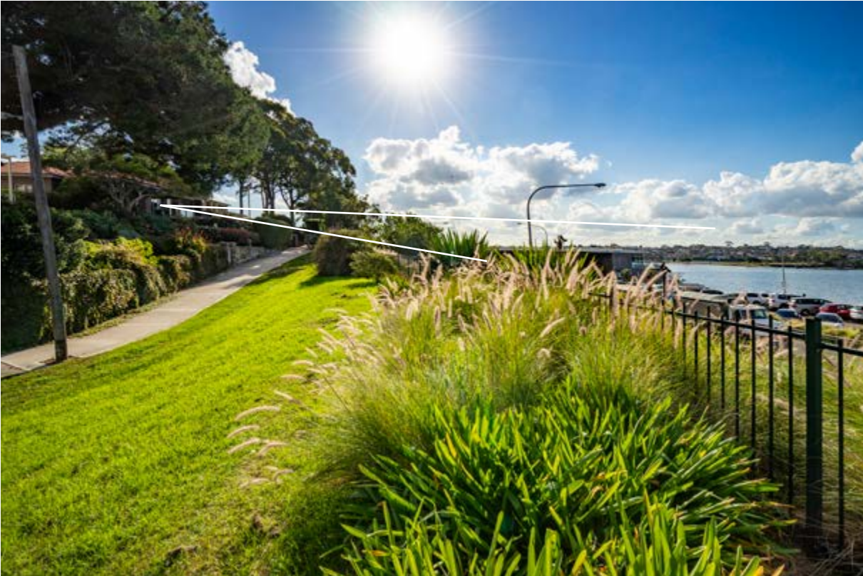
A noise mound integrated into the landscape ensuring views of the water but effectively blocking noise from the road.
