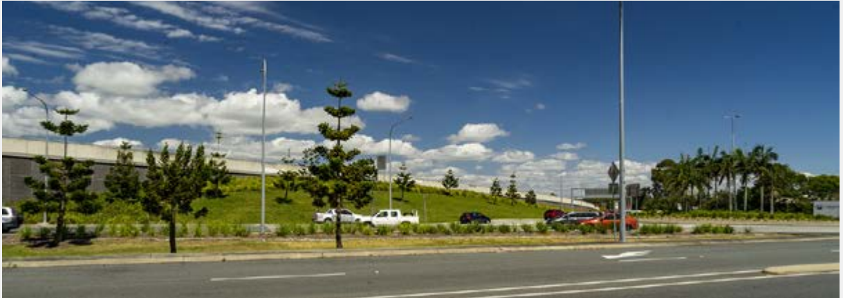
The Tweed Heads entrance from the Pacific Highway marked by pine trees, palms and a refined road infrastructure utilising dark tinted concrete panelling contrasting with the road parapet and breaking down the impact of the walls.
