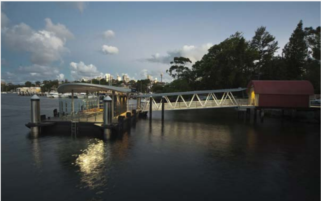
Balmain Wharf at Thames Street. The heritage shelter was retained as part of the ferry wharf design and creates a fitting gateway to the wharf in keeping with the character of the area.
