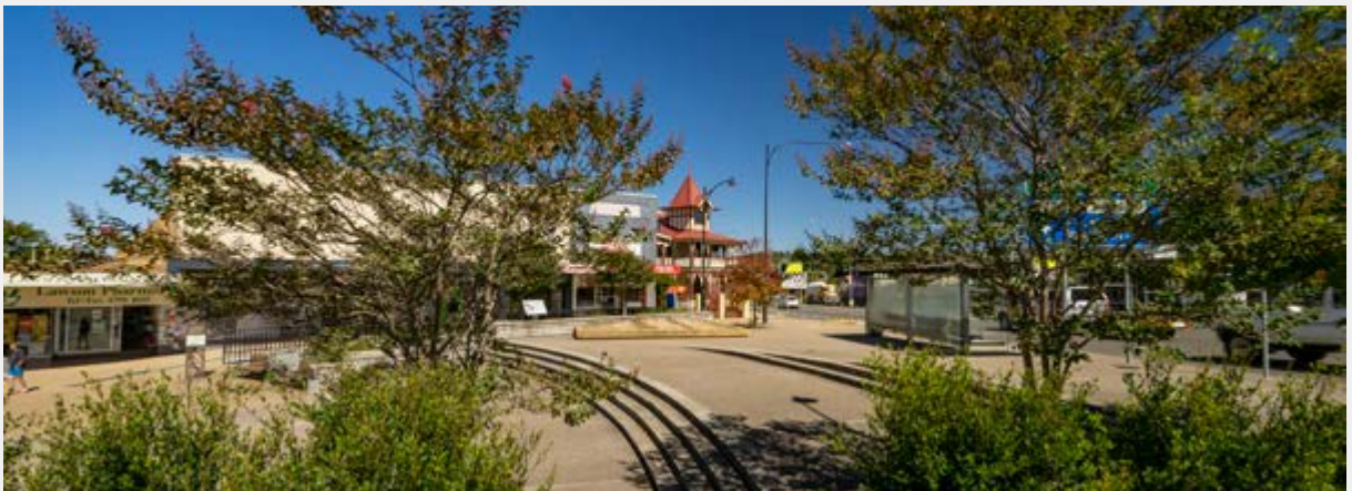
Lawson Douglass town centre revitalised and separated from traffic as part of the Great Western Highway Upgrade
