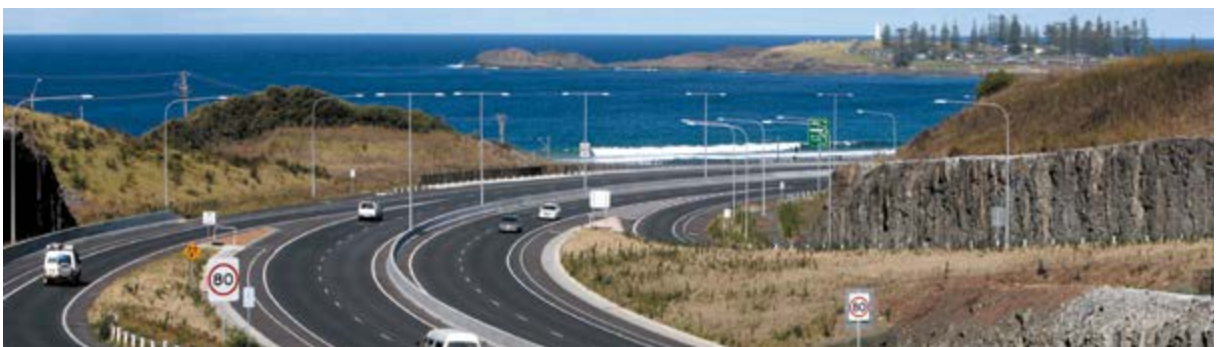
The approach to Kiama takes in views of Kiama itself, the Pacific Ocean and the beach at Bombo. The alignment of the edge of the quarry provided opportunities to steepen cuttings. Local dry stone walling was used at many locations on the project.
