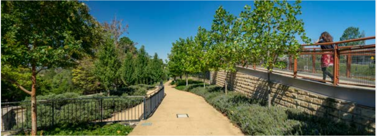
Memory Park was retained and improved in the upgrade works to the Great Western Highway at Hazelbrook. The park provides a reflective space for people shielded from noise below the corridor alignment.
