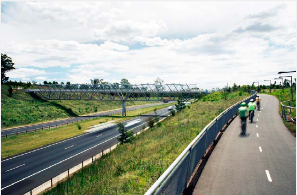
M7 shortly after opening in 2205 with the new landscape still in the establishment period. (Photograph by Roger D'Souza)
