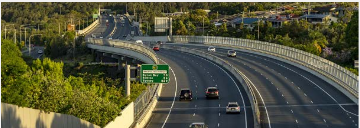
The view from the land-bridge looking south. The viaduct noise walls are clear acrylic to allow views and light and minimise visual impacts form properties.
