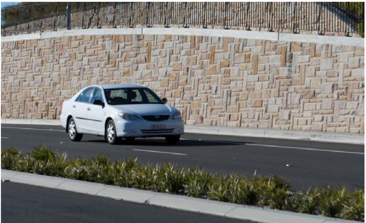
The use of sandstone in the retaining walls on the Great Western Highway provides a high quality context sensitive outcome
