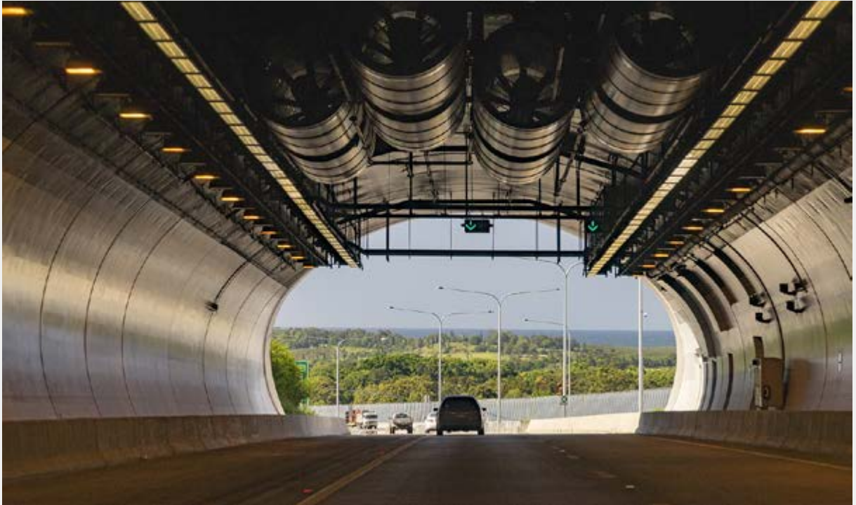
The view from the tunnel portal heading north frames the view of Cape Byron.
