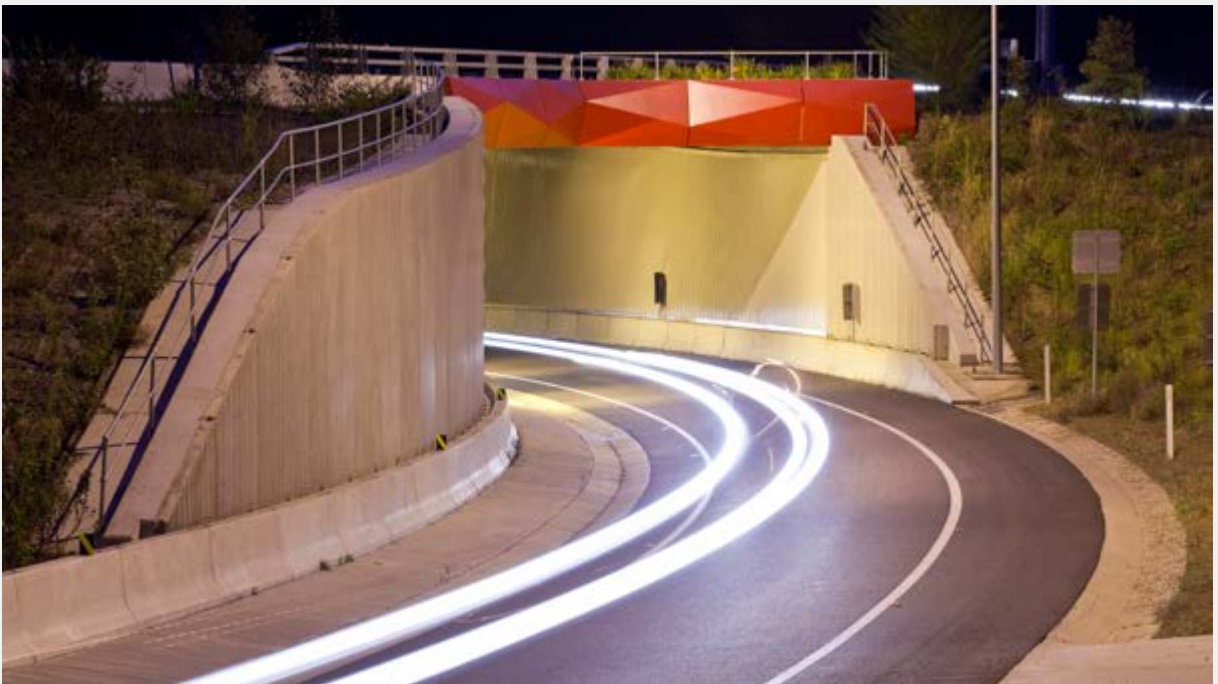
The Hunter Expressway utilised the bridge and underpass elements to accentuate the change in character along the route. Wall type abutment bridges were used rather than 'spill through' abutments to help create gateways or portals between one landscape character area and another. (Photo Greg Jackson)
