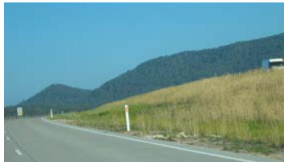
Karuah Bypass: Independently grading the carriageways helps minimise earthworks, provides a more interesting journey and reduces the wide terraced effect of roads on hillsides. Note the gentle gradient of the embankment.
