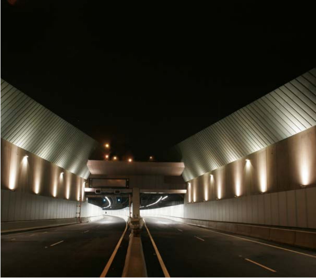
Lane Cove Tunnel eastern portal just prior to opening. The tunnel provided a four lane bypass of Epping Road and the Lane Cove area and completed the Sydney orbital motorway.
