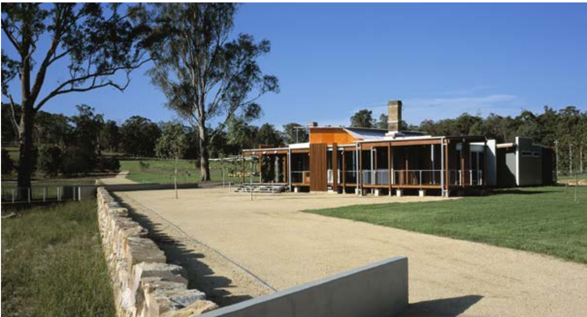
At Plough and Harrow Park, built as part of the M7 project, the old farm sheds were adaptively reused as a restaurant and café. The former Roads and Maritime worked closely with National Parks and Wildlife Services who managed the park and the lease for this building (picture Richard Glover).
