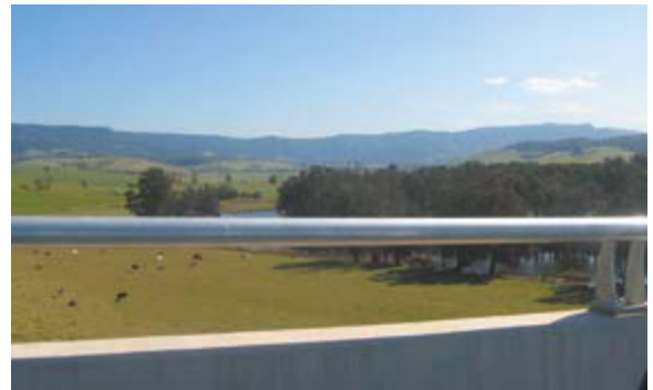
The bridges and barriers are designed to allow panoramic views of the Illawarra escarpment.
