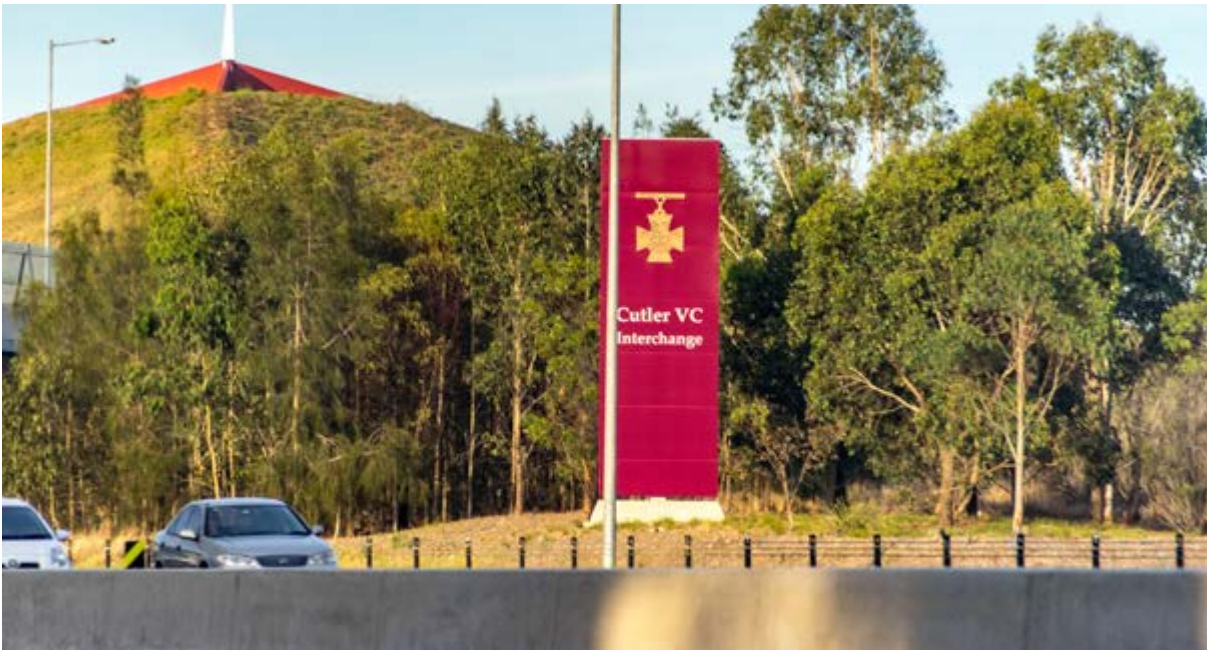
The Sir Roden Cutler Interchange marks the intersechange of the Remebrance Driveway and the M7. The marker posts highlight this place helping in wayfinding. The pyramid and finial detail is unique to this place.
