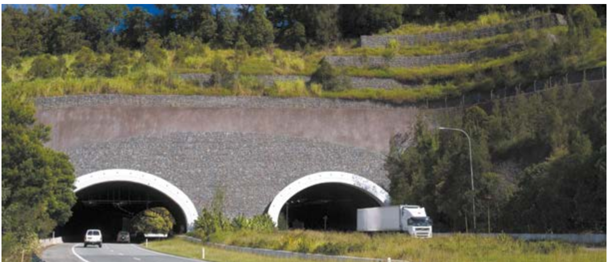
The Cudgen Road tunnel allows the wooded ridge line and wildlife corridor to cross the road and extend down to the edge of the Tweed River. Native planting and seeding is provided to revegetate the edges of the portal. Use of gabion facing is suitable for the natural context.
