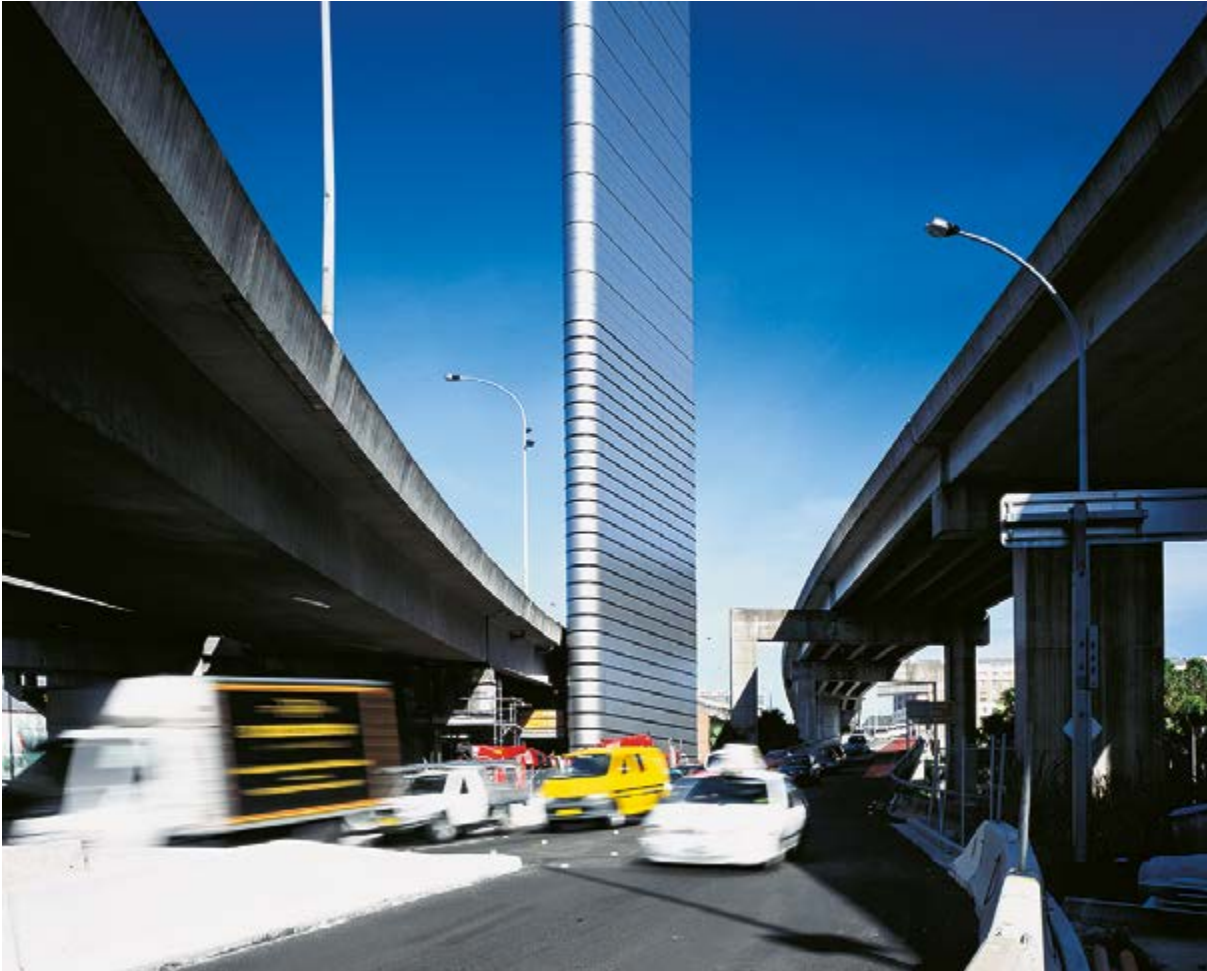
The ventilation outlet for the Cross City Tunnel fitted well into the architecture of the city at this location with a backdrop of skyscrapers and modern structures. Its slender design further minimises its impact in a beautiful way. (Photo Patrick Bingham-Hall)
