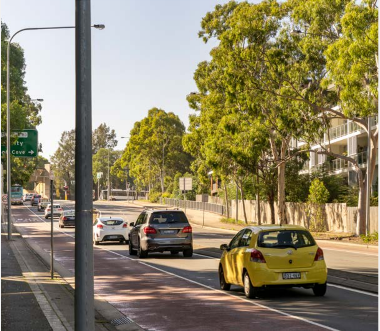
Epping Road realigned after the tunnel opened to accommodate better bus and active transport.
