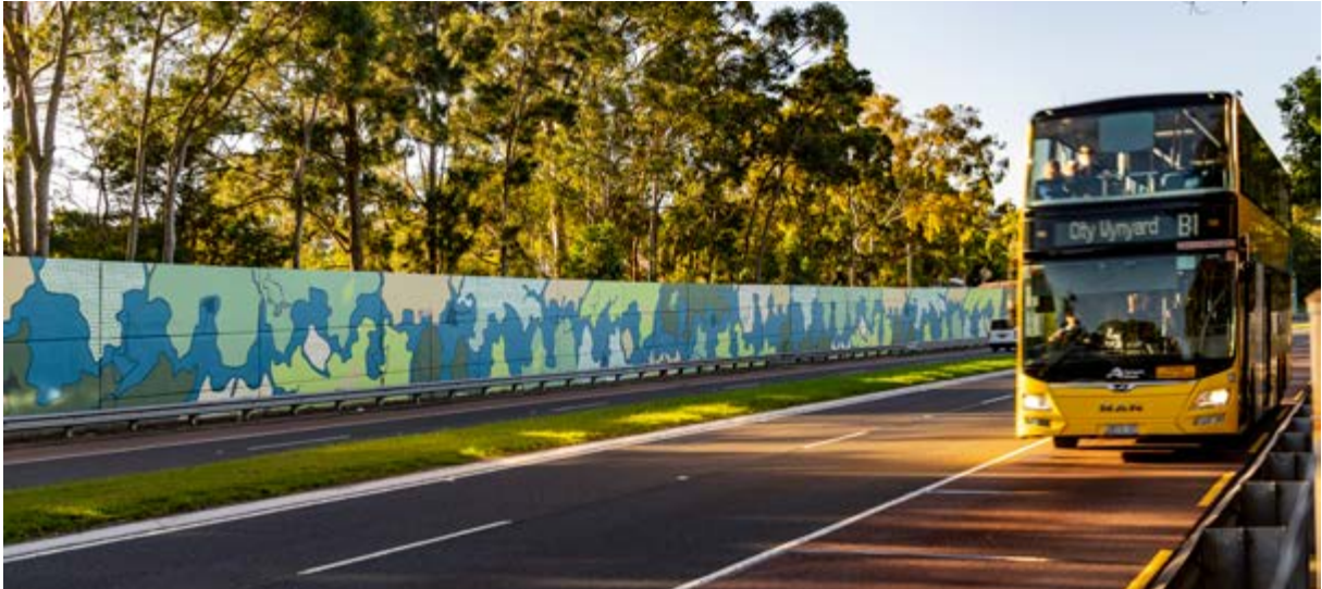
Shorelines and Storylines, an artwork on the noise wall at Burnt Creek deviation, was created by Balarinji Aboriginal Design and Strategy Studio in collaboration with the late Jessica Birk, a locally connected Aboriginal artist.
