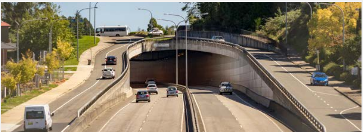
The Great Western Highway upgrade at the historic Blue Mountains town of Leura was set below the grade of Leura Mall allowing a 110m wide land-bridge, minimising traffic noise, creating views and forming a sensitive continuation of the main street.
