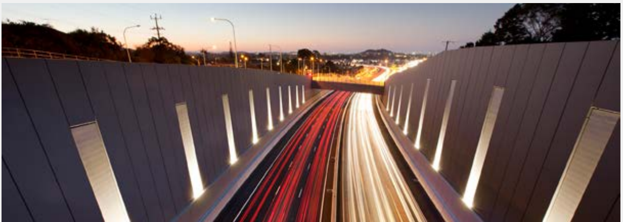
The Banora Point cutting from the land-bridge looking north to the Gold Coast. The retaining walls extend beyond the original surrounding ground plane to neatly provide the noise walls. Lighting is integrated into the walls to break down their expanse and create a night-time effect.
