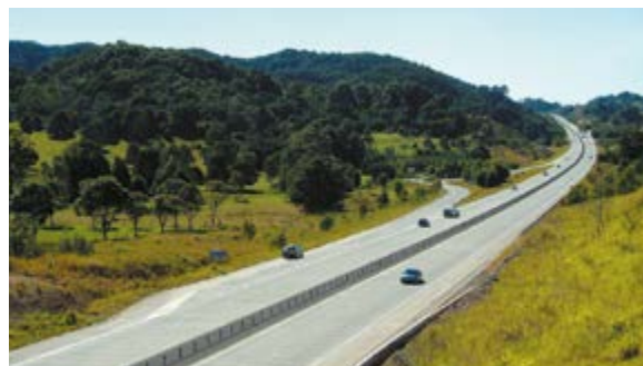
Yelgun to Chinderah: Avoiding cutting through spurs and aiming for saddles and valleys reduces earthworks and creates a more flowing, responsive alignment.
