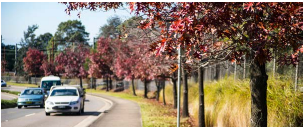
Pin Oaks were used on the Great Western Highway Upgrade at Faulconbridge. They were safely set back behind the required clear zone for the designed and posted 60km/h highway. They create a seasonal impact on the journey as well as a marker for the town and the different driving conditions.
