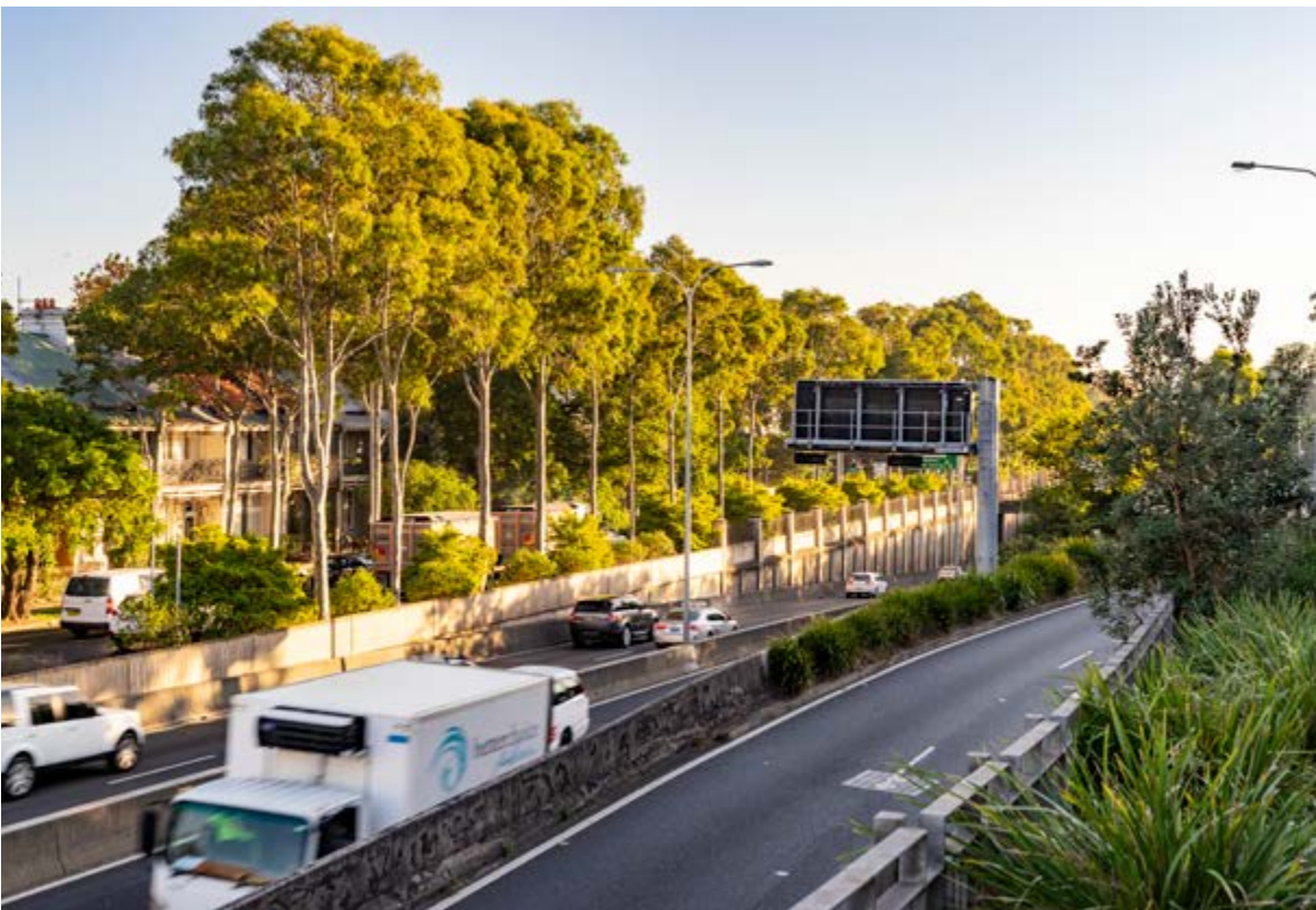
The Eastern Distributor was set down into a trench, minimising visual and noise impacts. Retaining walls ensured a minimal footprint and were designed to respond to the Victorian Terrace architecture on South Dowling Street.
