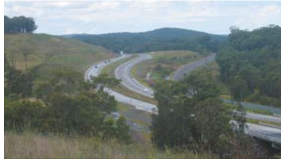
Karuah to Bulahdelah: Rounding off and grading out the slopes to 1:4 create an almost seamless integration with the natural slopes.
