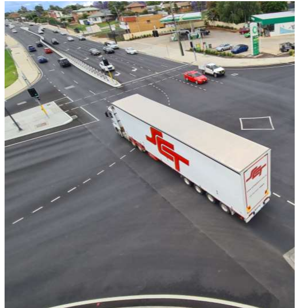
Newell & Mitchell Highway intersection upgrade
