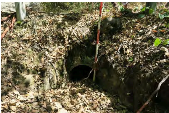
Figure 29. Site 9, culvert 357111 and dry stone headwall with evidence of concrete additions. Source: Extent Heritage, March 2023.
