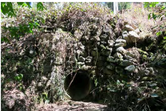
Figure 13. Site 3, culvert and dry stone headwall at chainage 120m, covered in vegetation. Source: Extent Heritage, March 2023.
