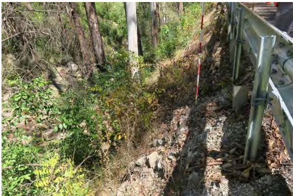
Figure 39. Site 13, remnant dry stone walls at chainage 20m, erosion along embankment, looking south. Source: Extent Heritage, March 2023.
