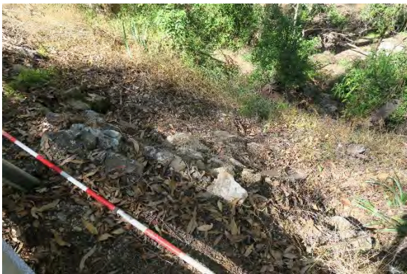
Figure 45. Site 13, dry stone wall at chainage 45-50m, erosion along embankment, looking downslope towards Darkey Creek. Source: Extent Heritage, March 2023.
