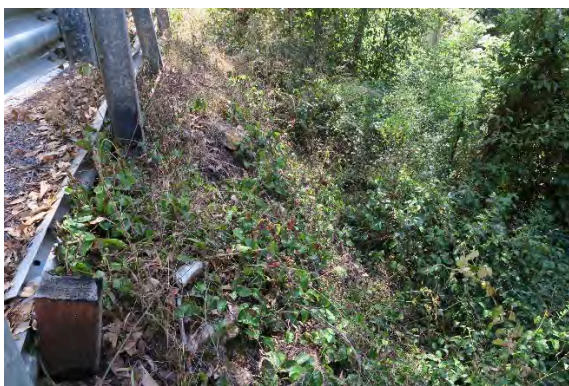
Figure 15. Site 4, remnant dry stone wall along eroded embankment, covered in heavy vegetation. Source: Extent Heritage, March 2023.
