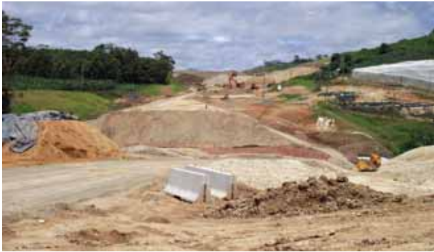
Earthworks near Greys Road on the Sapphire to Woolgoolga Upgrade, January 2011.
