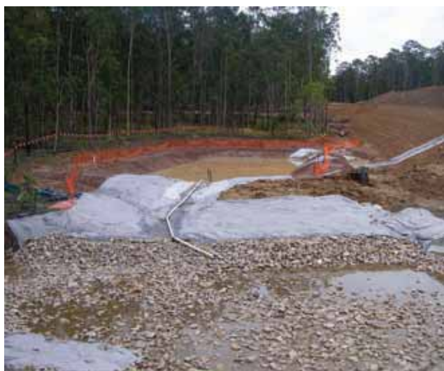
Dewatering a sediment basin via siphoning on the Pacific Highway Upgrade at Glenugie.
