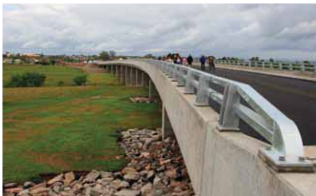
The completed Third Crossing of the Hunter River at Maitland, including the Harry Boyle Bridge, December 2010.
