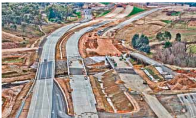
Aerial view of the Tarcutta Bypass, June 2011.
