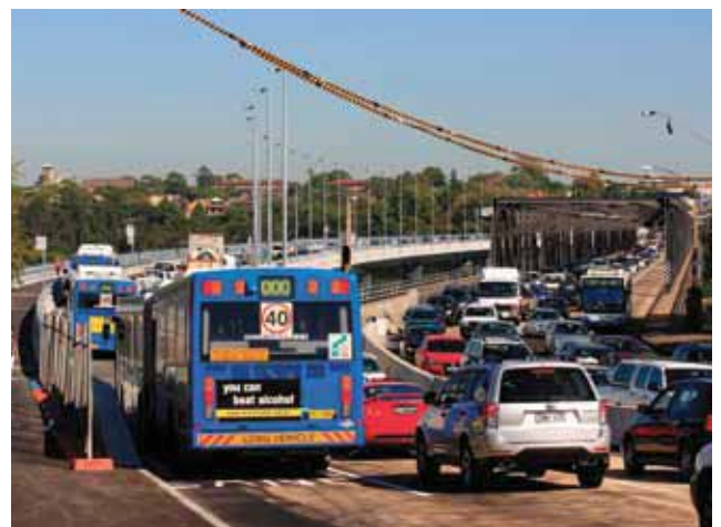
The completed $175 million Inner West Busway, January 2011.
