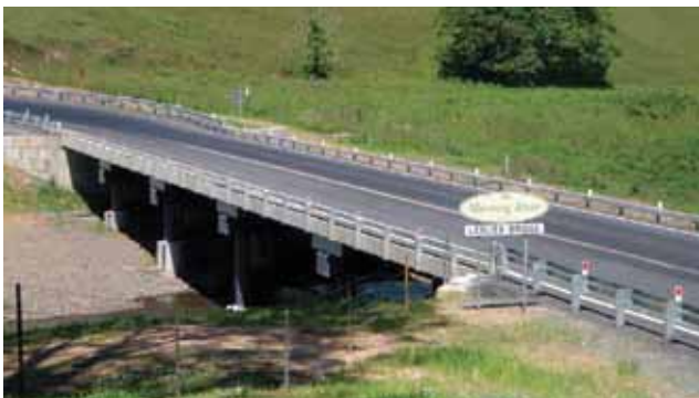
New Leslie's Bridge, Manning River, completed under the Timber Bridge Partnership, December 2010.
