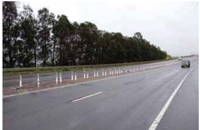
Wire rope safety barriers on the New England Highway at Maitland, November 2010.
