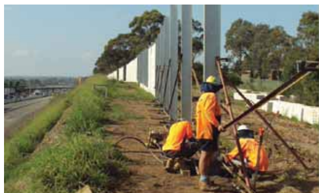
Construction of noise wall on the F5 Freeway, November 2010.
