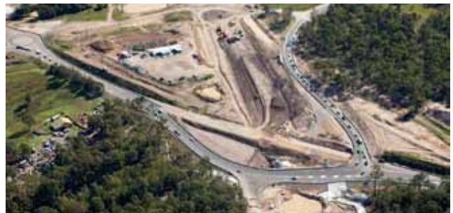
Aerial view of the Buchanan Interchange, Hunter Expressway, May 2011.
