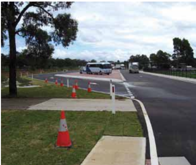
The Pheasants Nest heavy vehicle rest area, completed in November 2010.
