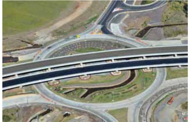
Teven interchange on the Ballina Bypass, May 2011.
