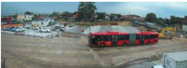
Work underway at Tempe bus depot for the State Transit Authority.
