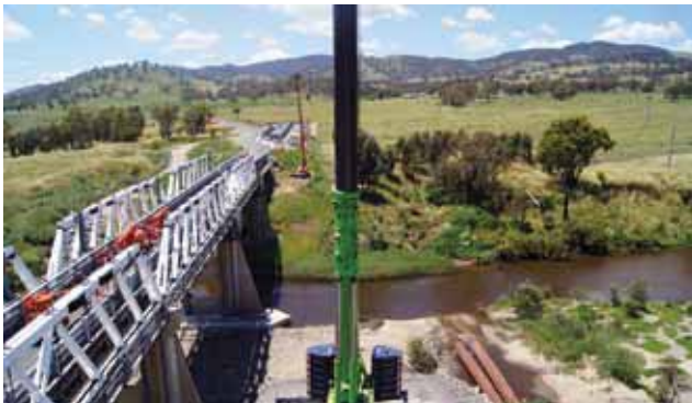
Restoration of the heritage-listed Tharwa Bridge, November 2010.
