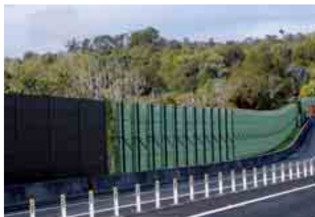
This noise wall along the Pacific Highway at Ewingsdale is just one of the measures the RTA uses to reduce highway noise.
