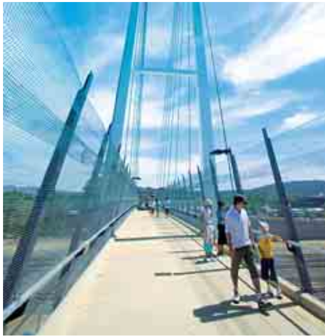
The Albury Wodonga Hume Freeway project opening was celebrated by more than 20,000 community members with a walk over the freeway before it opened to traffic.
