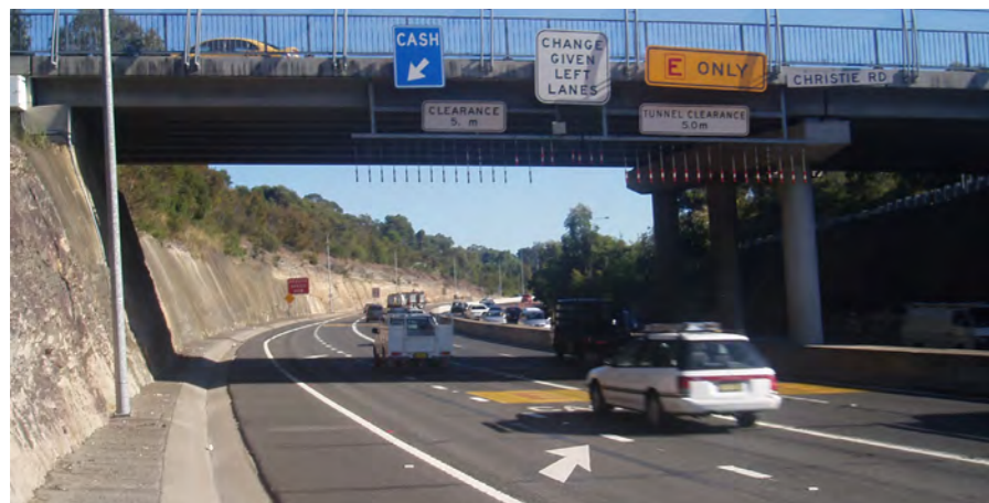
Photo 6.2.12 Christie Road Overbridge.
