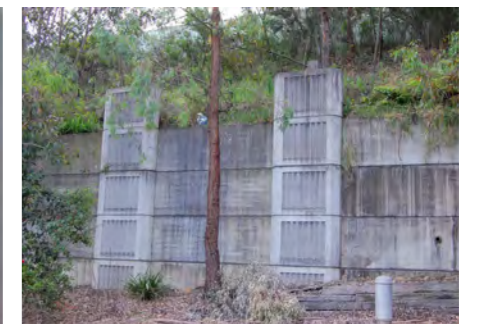
Photo 6.2.15 Existing wall facing Junction Road
