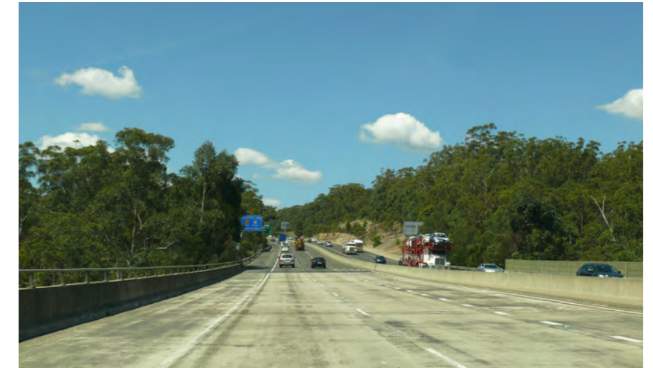
Photo 3.24 View of existing motorway environs crossing Darling Mills Creek.
