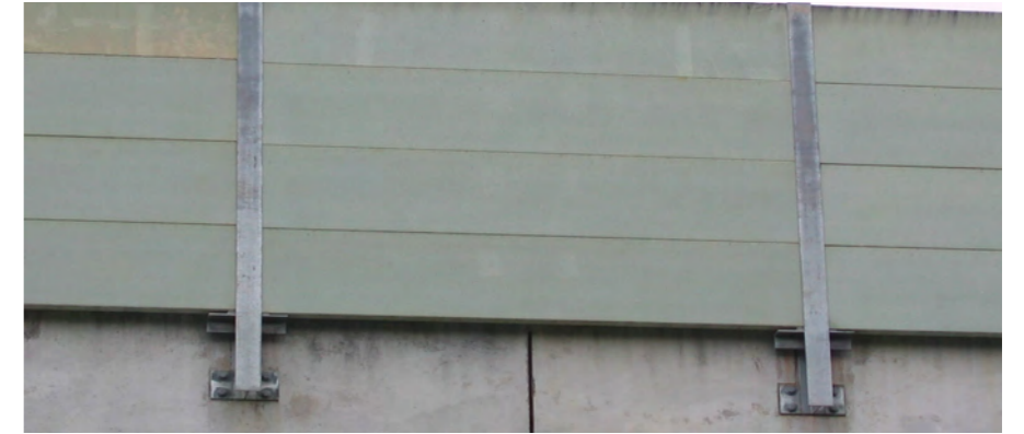
Photo 5.28 Solid noisewalls fixed to the bridge parapets at Khartoum Road.
