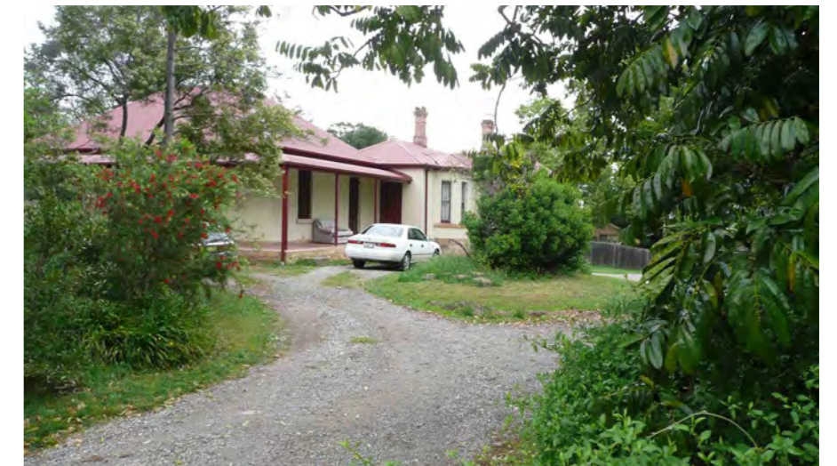
Photo 3.16 View of Heritage Homestead 266 Windsor Road
