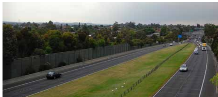
Photo 2.26 Precinct 1 - Western view from Windsor Road
