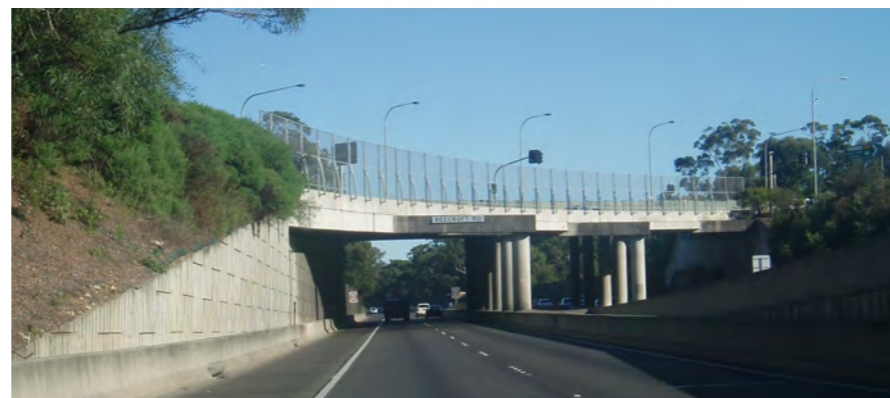
Photo 5.22 Bridge at Beecroft Road with exposed piers and headstocks.
