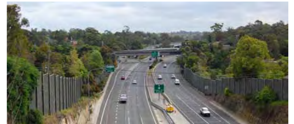
Photo 2.28 Precinct 3 - Western view from the top of Norfolk Road tunnel portal
