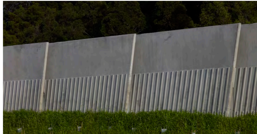
Photo 5.5 Patterned precast concrete panels on the Pacific Highway.
