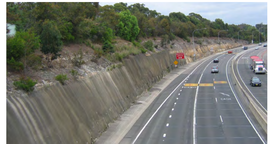
Photo 5.16 Shotcrete stabilisation applied to a near vertical cutting.
