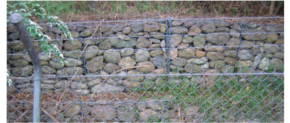
Photo 5.35 Low gabion basket walls near Khartoum Road bridge.
