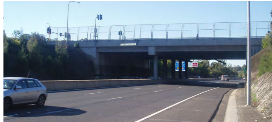
Photo 5.20 Lane Cove Road double span overbridge.
