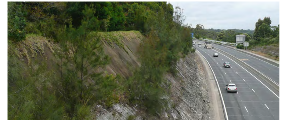
Photo 5.19 Shotcrete stabilisation and vegetation on top of a cutting.
