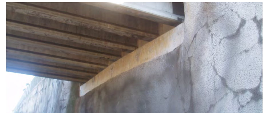
Photo 5.37 Shotcreted abutment cutting at Watkins Road overbridge.
