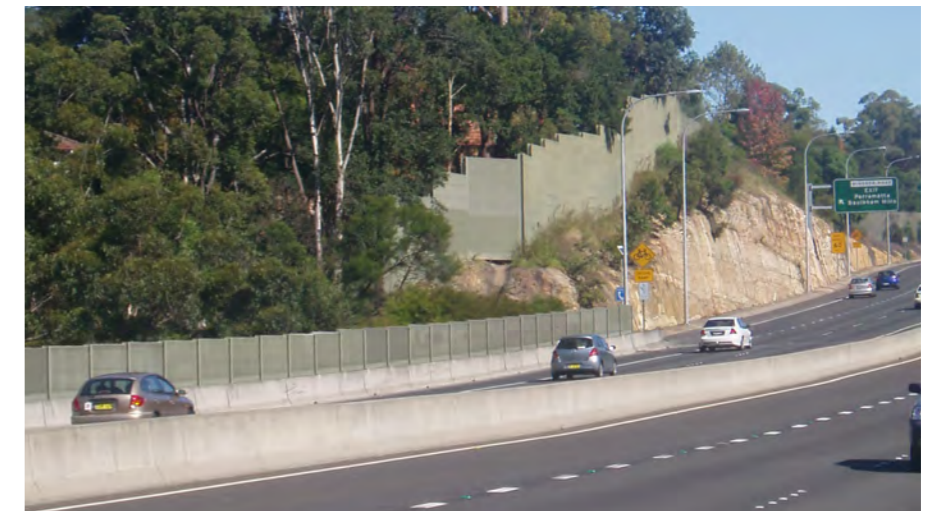
Photo 5.4 Noisewalls with irregular stepping and offset from the road edge.
