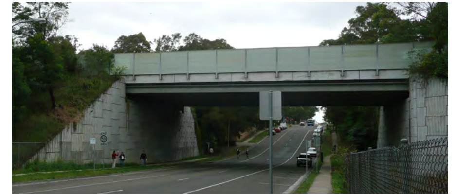
Photo 5.24 Noisewall adds extra depth to the structure over Khartoum Road.
