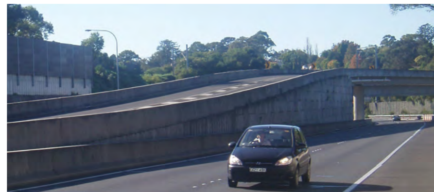
Photo 5.34 Precast concrete walls at Beecroft Road bus ramps.
