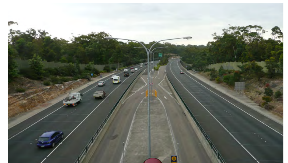
Photo 3.26 View from Barclay Road Bridge and abutment.
