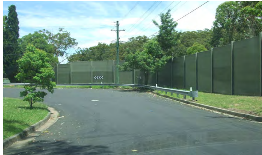
Photo 3.21 View of existing noise wall adjacent Carmen Drive.
