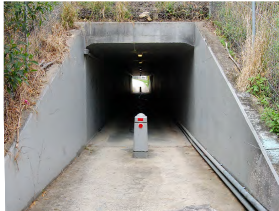
Photo 6.2.9 Vimiera Road Pedestrian Underpass
