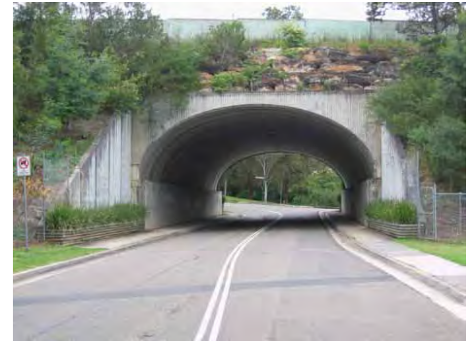
Photo 2.22 "Bebo" arch bridge over Busaco Road
