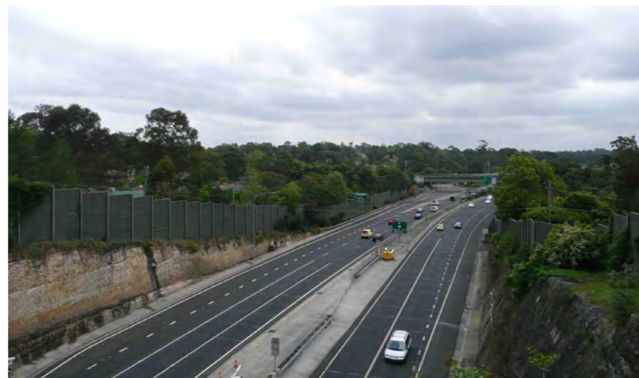
Photo 3.5 Precinct 3 - View from Western Tunnel Portal to Beecroft Road.
