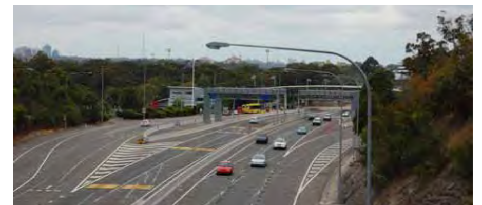
Photo 2.9 Toll plaza located on the broad flat ridge
