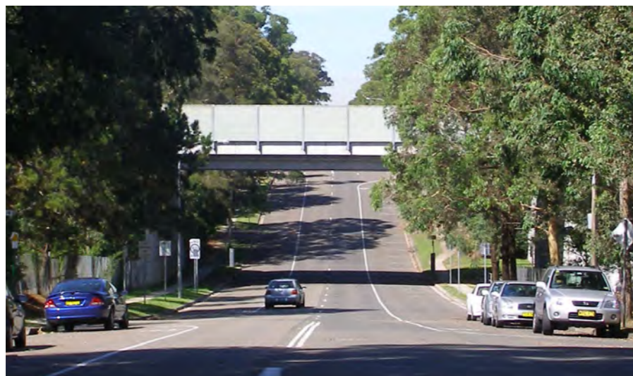
Photo 6.2.13 Khartoum Road Overbridge.
