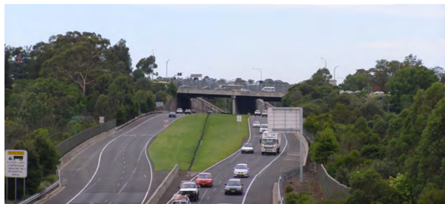
Photo 6.2.1 Looking East towards Windsor Road Interchange
