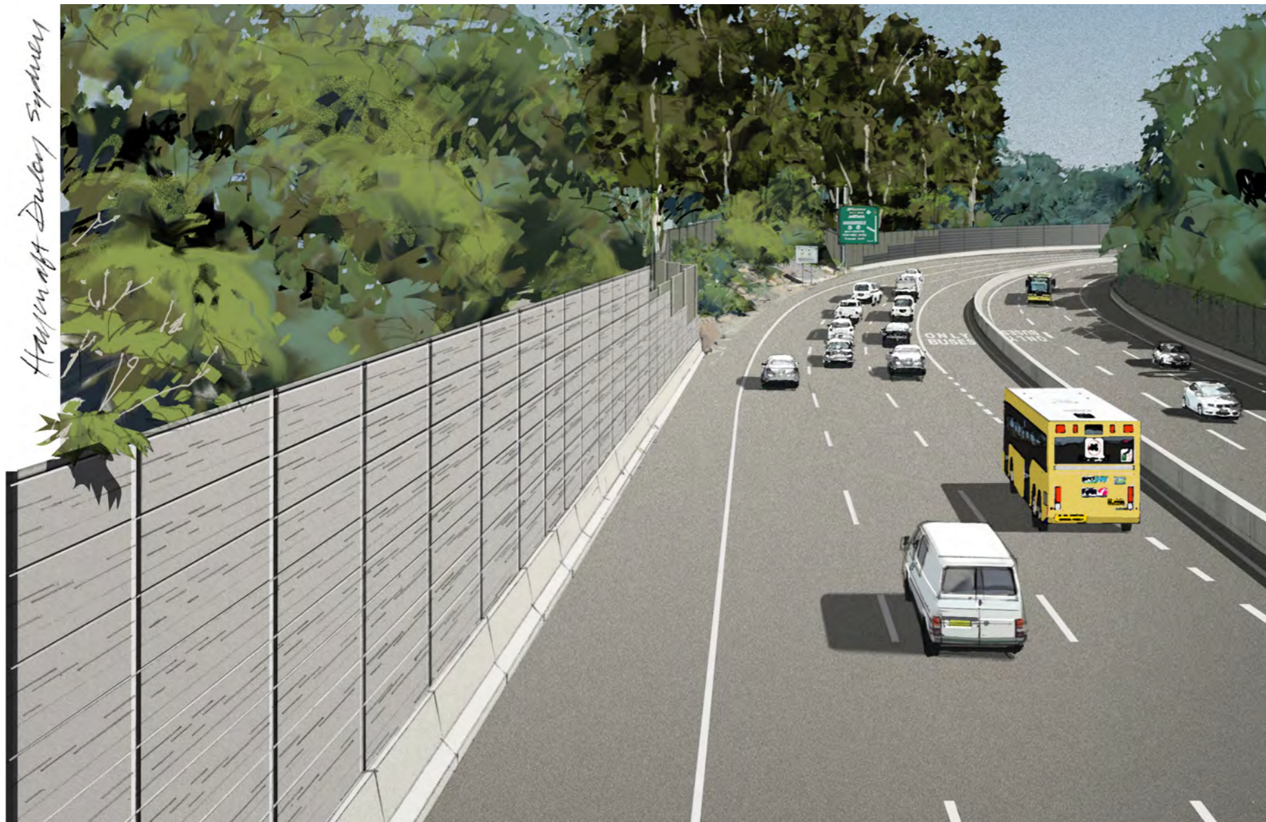
Figure 6.2.33 Perspective showing insertion of new Type H wall with existing noise walls.
