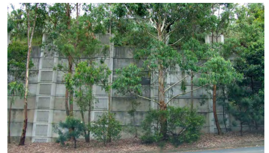
Photo 3.13 Existing noise wall and screen planting on Junction Road.
