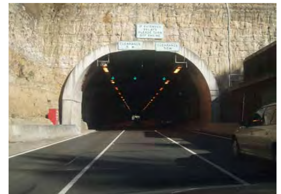
Photo 2.12 Tunnel portal area reveals the local geology
