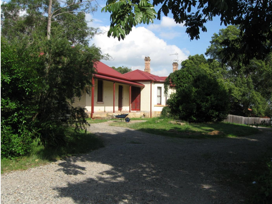
Figure F6: View of 266-268 Windsor Road showing bay window. View south west.
