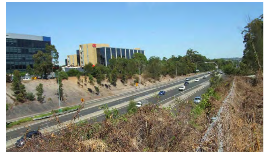
Photo 3.9 Precinct 5 - View from Lane Cove Road looking west revealing shale cutting and the office development beyond.
