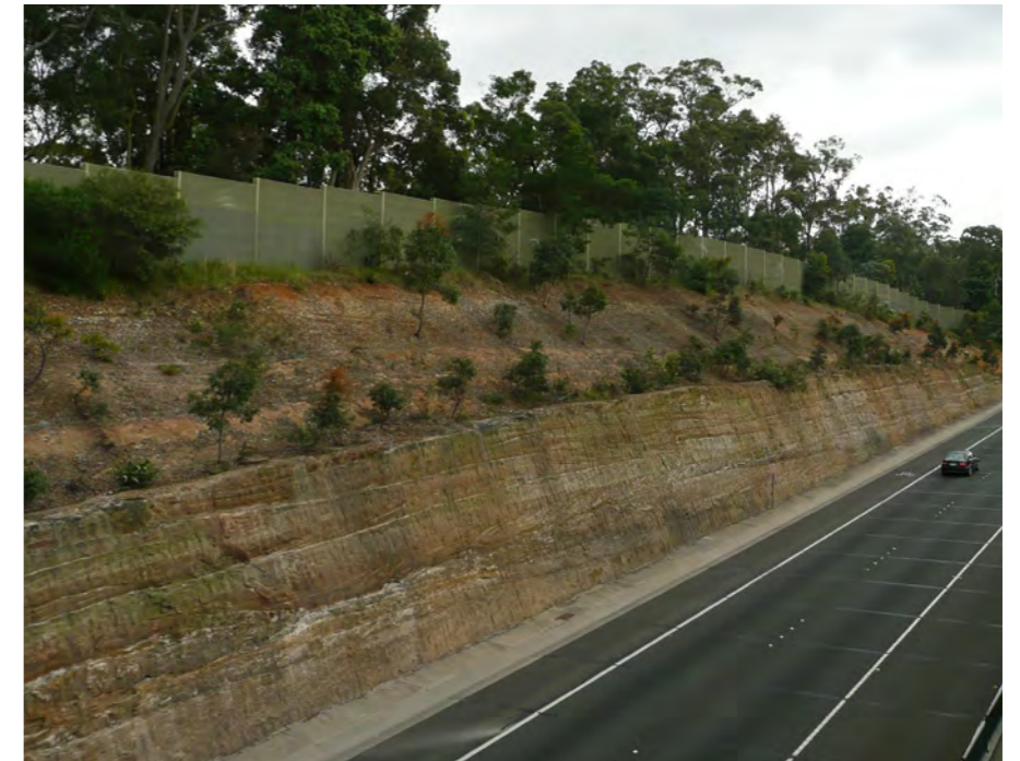
Photo 5.15 A near vertical cutting without benching.
