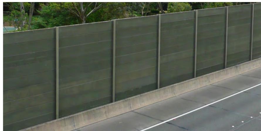
Photo 5.6 Hebel wall with clean lines and top edge.
