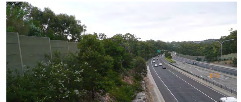
Photo 5.18 Revegetation of a cutting conceals the noise wall.
