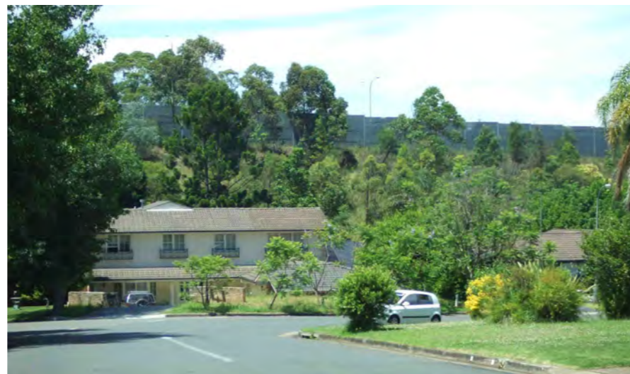
Photo 3.23 View of noise wall adjacent to east bound off ramp from Westmore Drive. No additional impacts to occur at this location.
