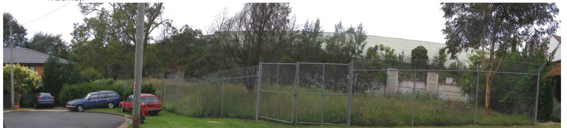
Photo 3.15 View from Craig Avenue to M2 Motorway retaining wall and noise walls.
