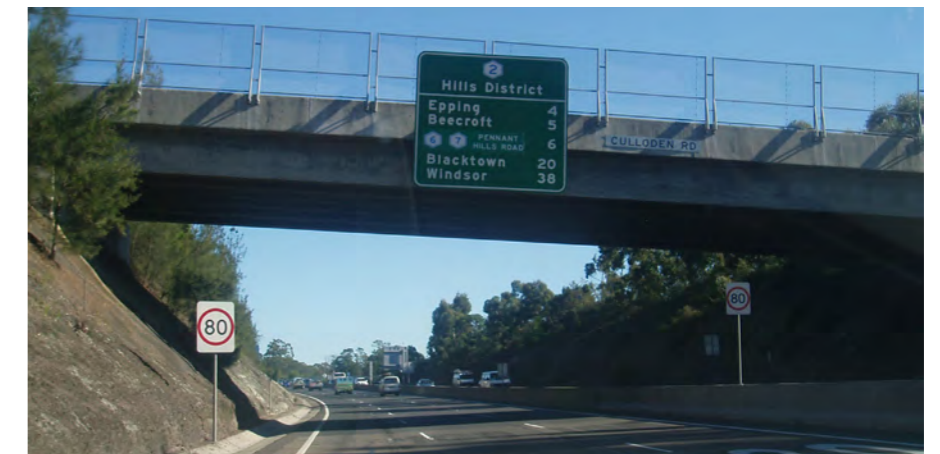
Photo 6.2.11 Culloden Road Overbridge
