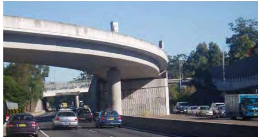
Photo 2.31 Bridge abutment at Beecroft Road Interchange
