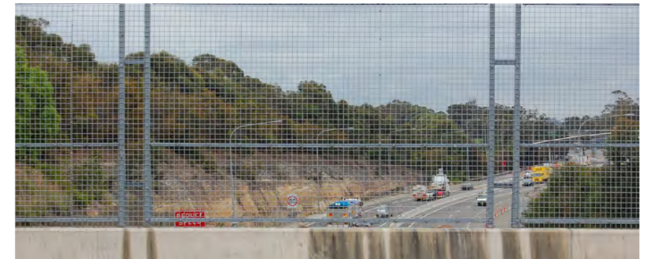
Photo 5.29 Simple, well defined safety screens on Christie Road overbridge.
