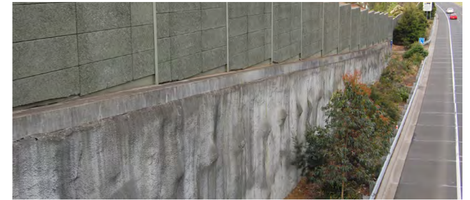
Photo 5.17 External rock bolts beneath shotcrete stabilisation.
