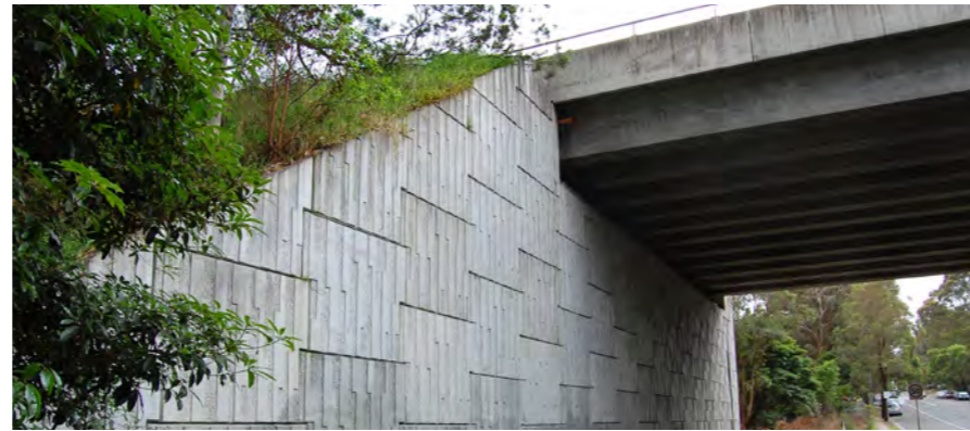
Photo 5.32 Precast concrete panel wall bridge abutment at Khartoum Road.
