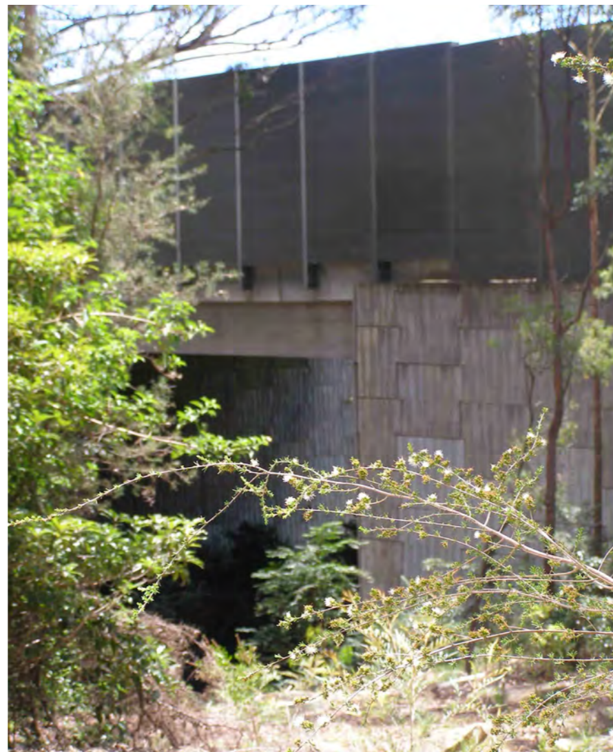
Photo 3.19 Close-up view of bridge from rear property boundary.
