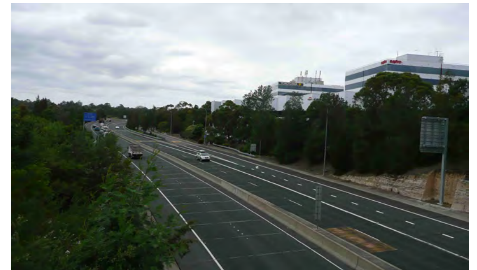
Photo 3.8 Precinct 5 - View from Herring Road towards Macquarie Park commercial.
