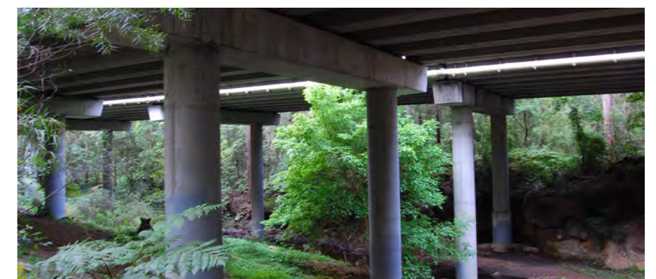
Photo 5.27 Double motorway bridge over bushland and Devlins Creek.
