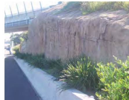
Photo 6.2.23 Better quality finish of coloured shotcrete used at Abbott Road Bridge
