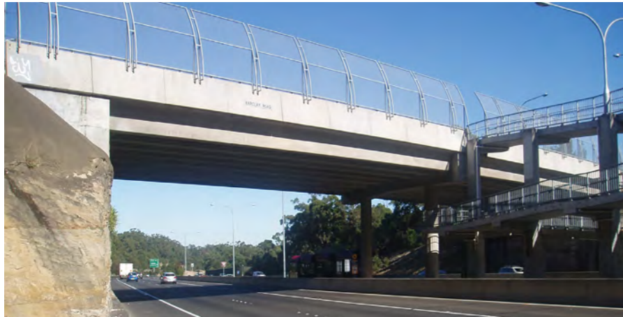
Photo 6.2.3 Barclay Road Overbridge
