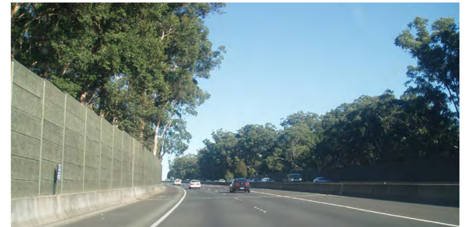
Photo 6.2.5 Devlins Creek Bridge
