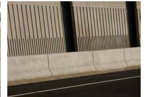
Photo 6.2.4.2 F Type Barrier
