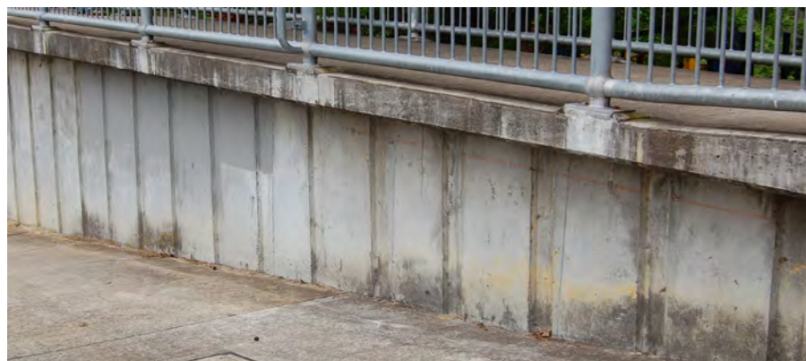
Photo 6.2.21 In-situ concrete wall at pedestrian overpass at Kent Street
