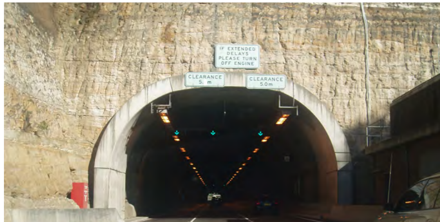
Photo 6.2.7 Eastern portal of the Norfolk Tunnel.
