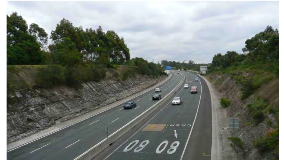
Photo 3.7 Precinct 5 - View from Christie Street bridge looking west.
