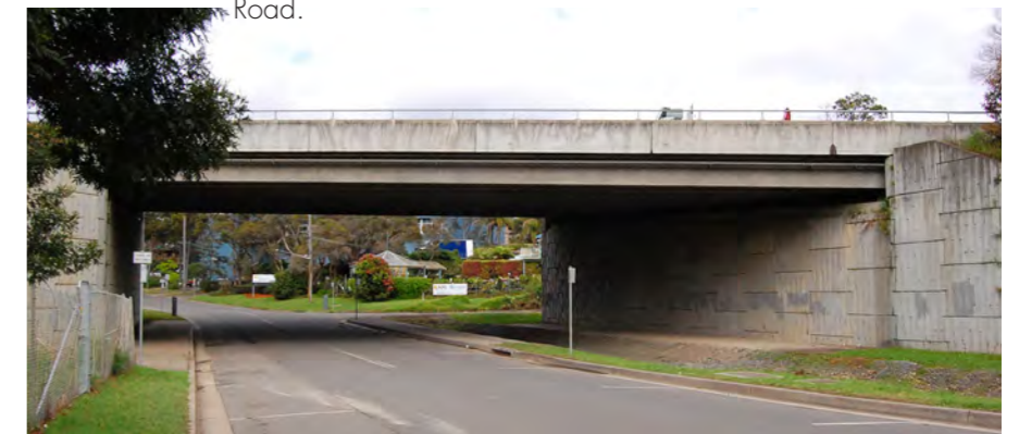
Photo 5.25 Single span Super-T girder bridge over Wicks Road.
