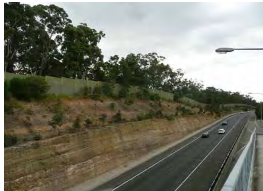
Photo 2.11 Sandstone is exposed in the motorway cuttings
