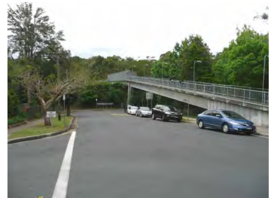
Photo 2.23 Pedestrian bridge near Epping Heights Primary School
