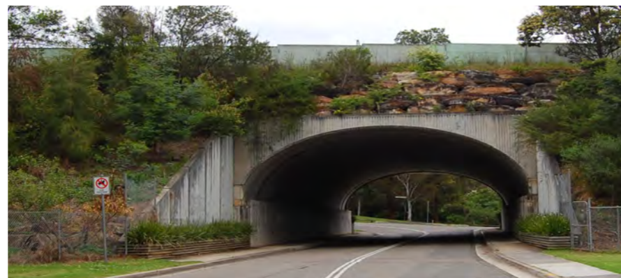
Photo 6.2.10 "Bebo" arch Bridge over Busaco Road
