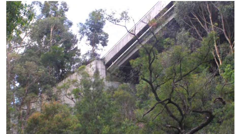
Photo 3.18 View of eastern abutment to Darling Mills Bridge.
