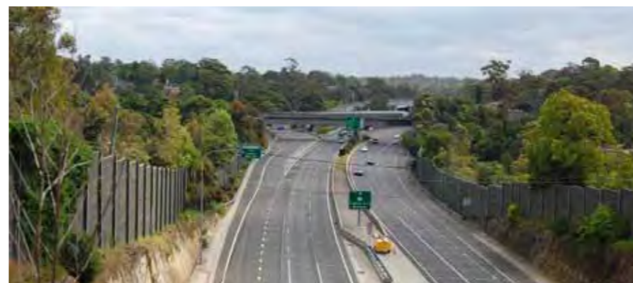
Photo 2.6 View west over Devlins Creek valley
