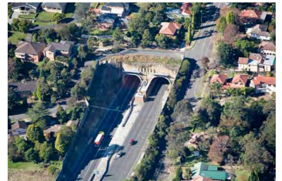
Photo 2.25 Sandstone cuttings and noise walls at the western Norfolk Road Tunnel portal
