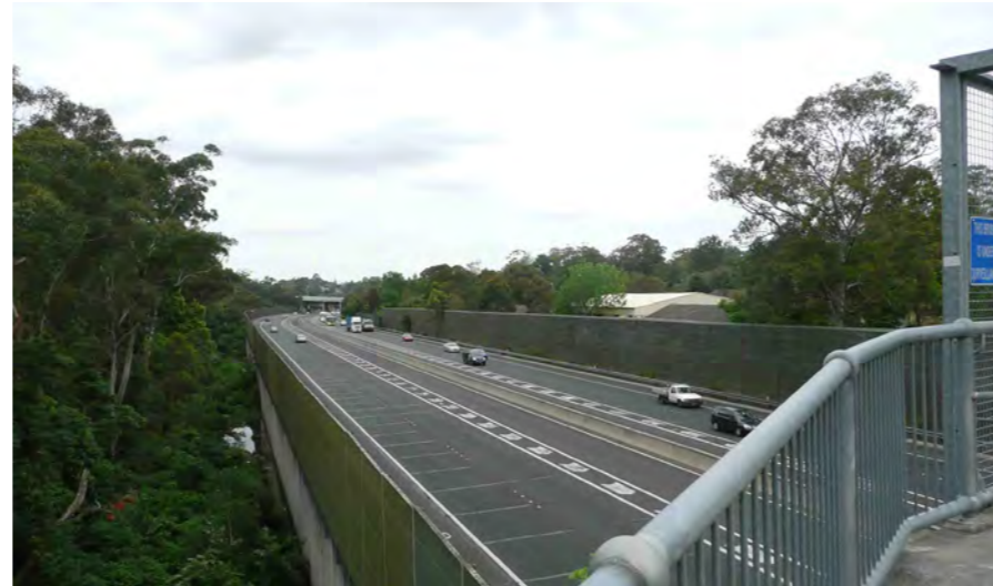
Photo 3.4 Precinct 3 - View looking east from Kent Street bridge showing walled corridor.
