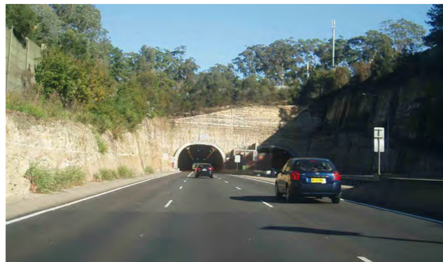
Photo 3.6 Precinct 4 - Eastern Tunnel Portal with sandstone geology exposed
