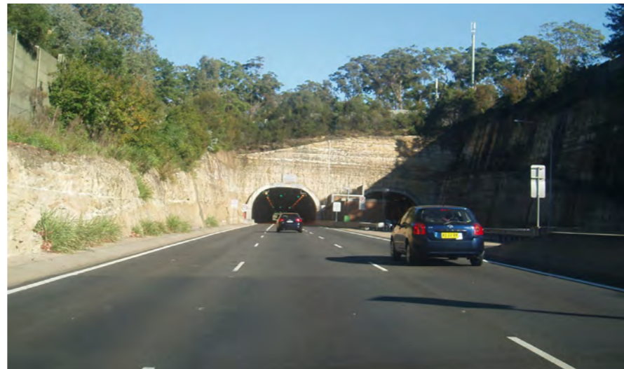
Photo 3.35 View of eastern tunnel approach.
