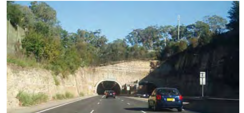
Photo 2.7 Eastern portal of Norfolk Road Tunnel
