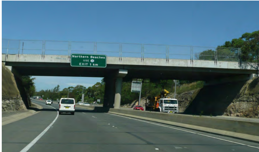
Photo 3.45 View of Christie Road Bridge and abutments.
