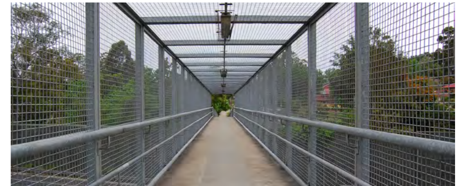
Photo 5.30 Well integrated handrails on the pedestrian bridge at Kent Road.
