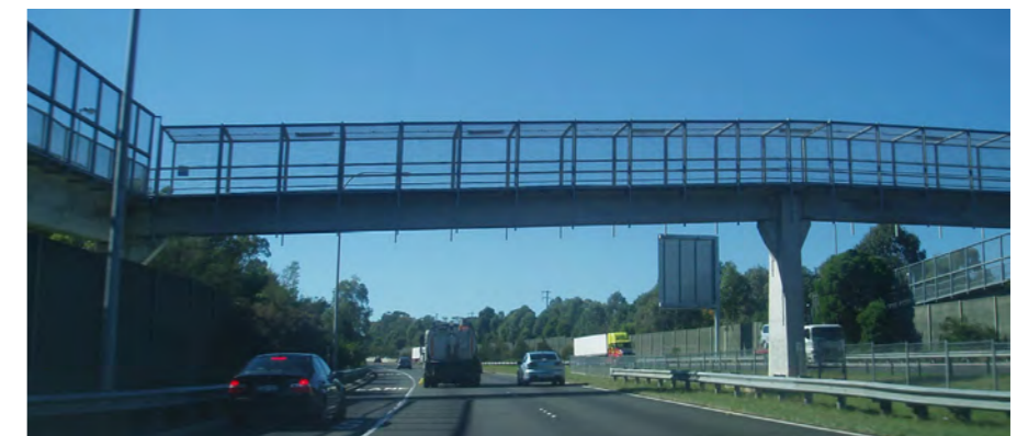
Photo 5.26 Pedestrian bridge over the M2 Motorway.
