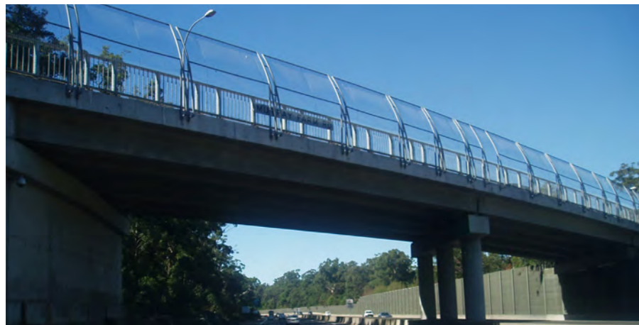
Photo 6.2.6 Kirkham Street Overbridge..
