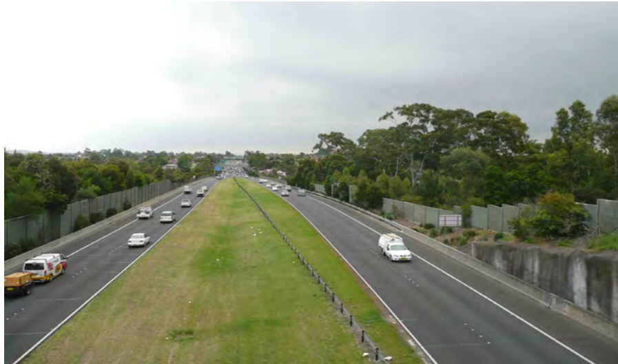
Photo 3.1 Precinct 1 - View from Windsor Road Overbridge reveals a corridor contained between noise walls.
