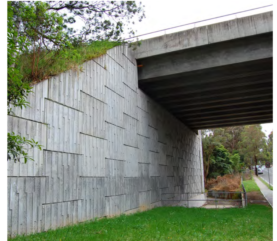
Photo 6.2.16 Wicks Road Bridge
