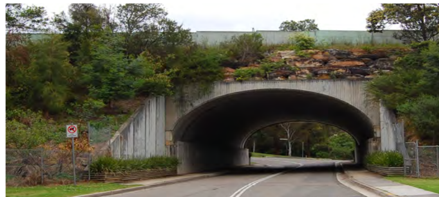
Photo 5.21 "Bebo" arch bridge over Busaco Road.
