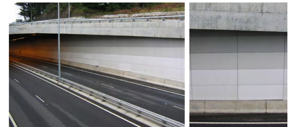
Photo 6.2.19 Compressed Fibre Cement Cladding Panels
