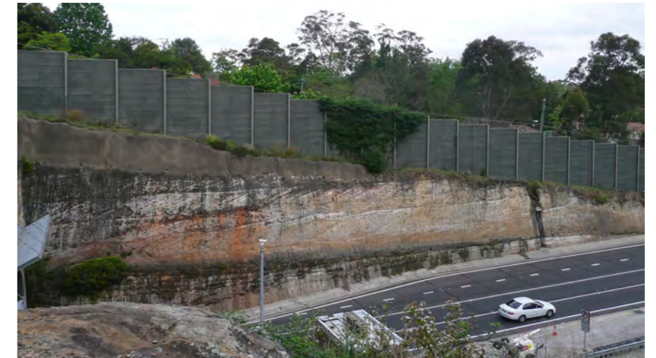
Photo 5.2 Sandstone cutting with shotcrete top edge and noisewall.
