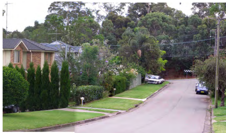
Photo 3.14 Murrills Crescent looking to embankment and noise wall of M2 Motorway.
