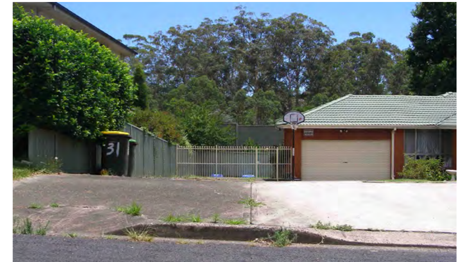
Photo 3.22 View of existing noise wall to the rear of property in Carmen Drive.
