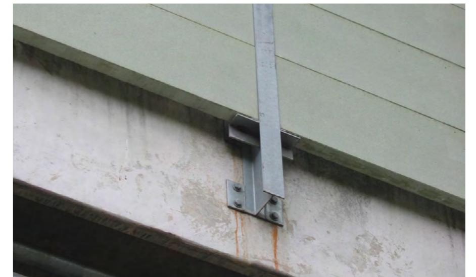
Photo 5.14 Noise wall post connection to a bridge parapet.
