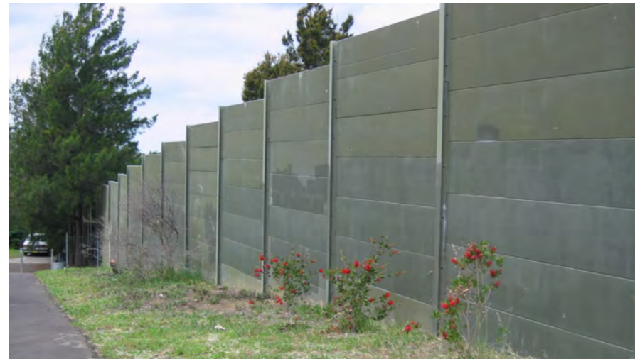
Photo 5.11 Noise wall posts viewed from the off-road side.
