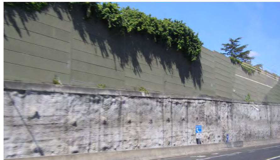
Photo 5.3 Noisewall on top of shotcrete wall at Pennant Hills Road Interchange.
