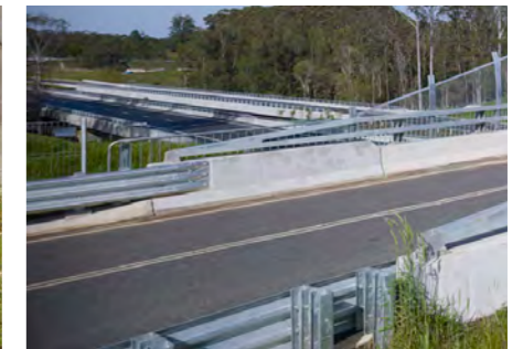
Photo 6.2.4.4 Thrie Beam Barrier
