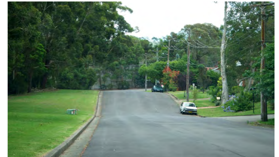
Photo 3.11 View from Godin Street to retaining walls of M2 Motorway.
