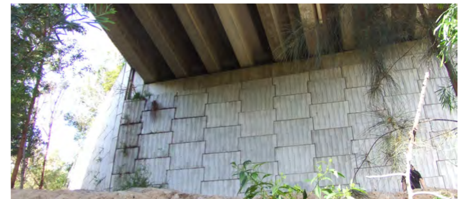
Photo 6.2.17 Terrys Creek Bridge
