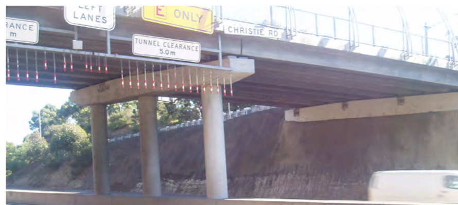
Photo 5.23 Piers and headstocks beneath Christie Road overbridge.
