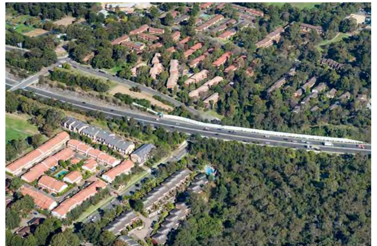
Photo 2.21 Medium density residential housing adjacent to the M2 Motorway at Marsfield
