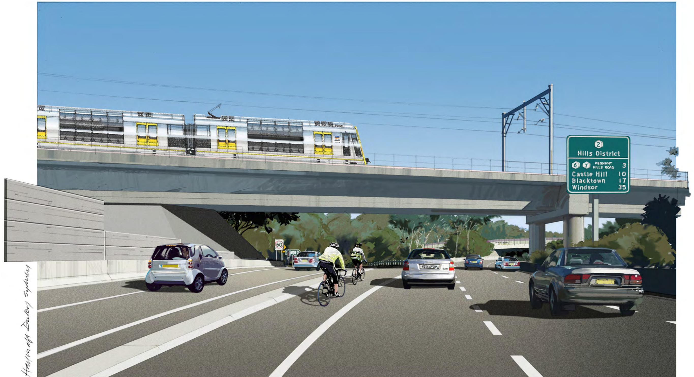
Figure 6.1.40 Artists perspective of Beecroft Road and Rail Bridge looking west (approximately Stn 12400) showing the removal of the bus lane bridge, cycleway on shoulder and new noise wall.
