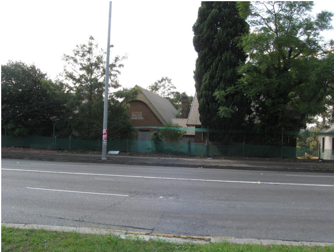
Figure F8: View from 266-268 Windsor Road showing Baulkham Hills Public School. View north
