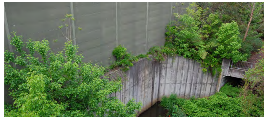
Photo 5.33 In-situ concrete walls along Devlins Creek at Kirkham Street.
