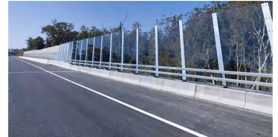
Photo 5.8 Transparent panels on a Pacific Highway bridge.
