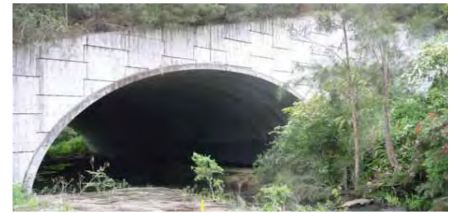
Photo 2.8 Bridge over Shrimptons Creek
