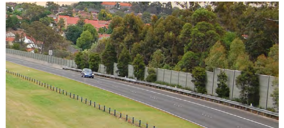
Photo 5.10 Poor and irregular planting between traffic barrier and noise wall.
