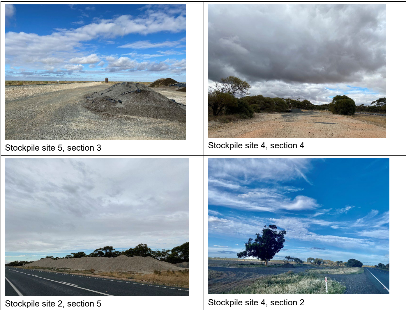
Figure 3-1: Examples of existing stockpile sites along the proposal length.
