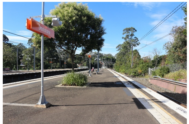
FIGURE 5-2 VIEW SOUTHEAST ALONG STATION PLATFORMS
