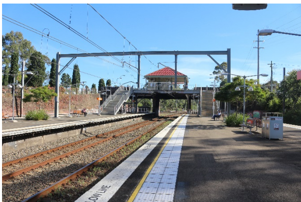
FIGURE 5-1 VIEW NORTHWEST ALONG THE STATION PLATFORMS
