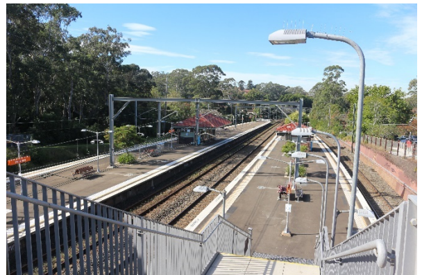
FIGURE 5-3 VIEW FROM THE ELEVATED STATION CONCOURSE, ACROSS THE STATION PLATFORMS
