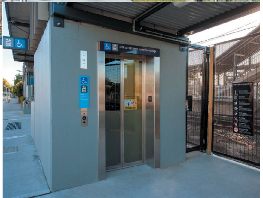
New lift at Canley Vale Station
