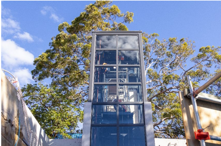
Lift on Como Parade looking up from rail underpass
