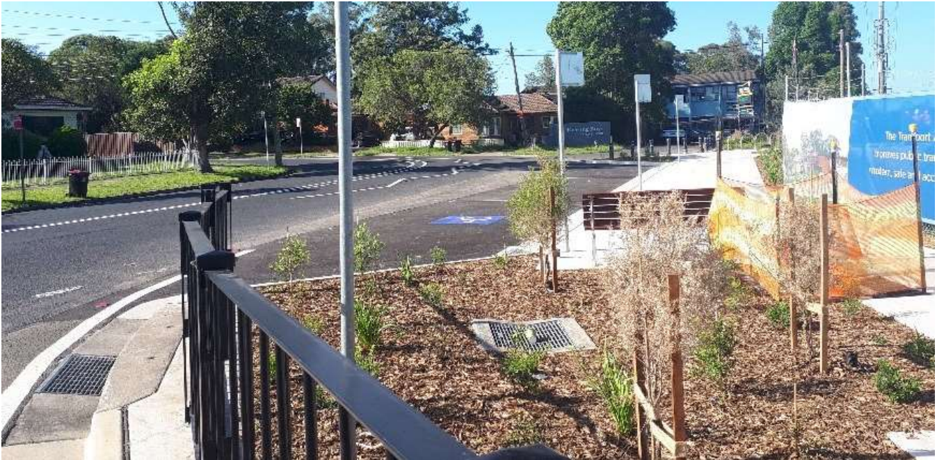
Completed work in Teresa Street, Birrong
