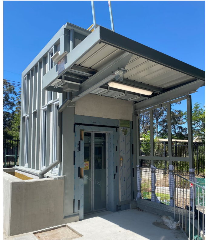
Pictured above: Lift construction progress at Beecroft Station, October 2021
