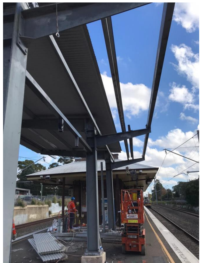
Removal of canopies during May weekend work
