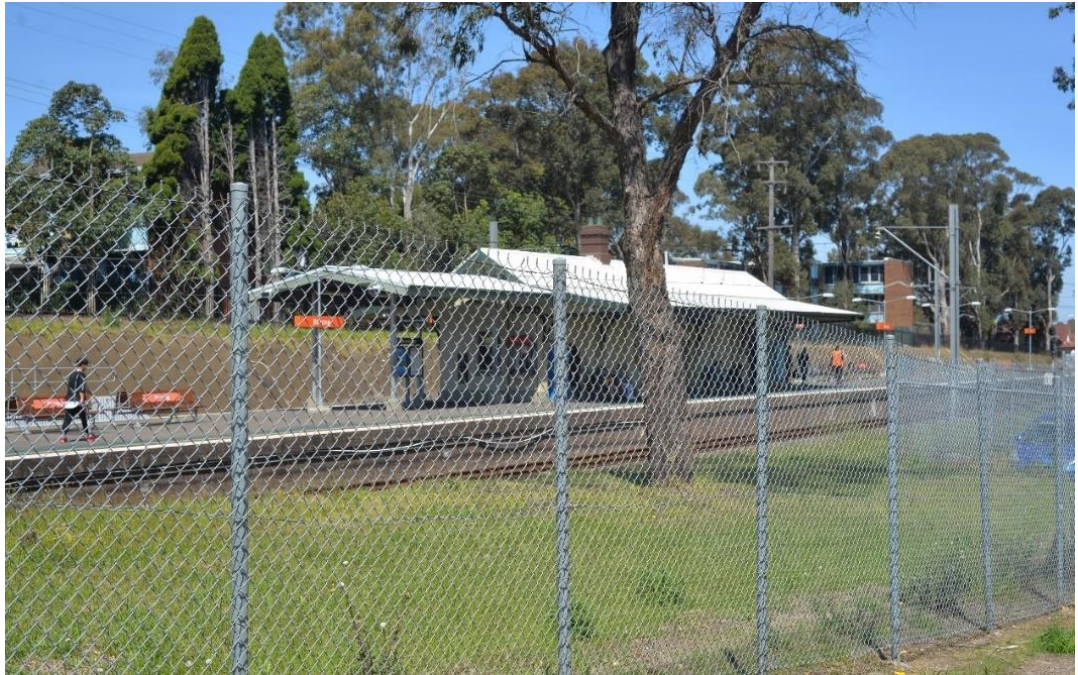
FIGURE 3-3: VIEW OF BIRRONG STATION BUILDING FROM HUDSON PARADE
