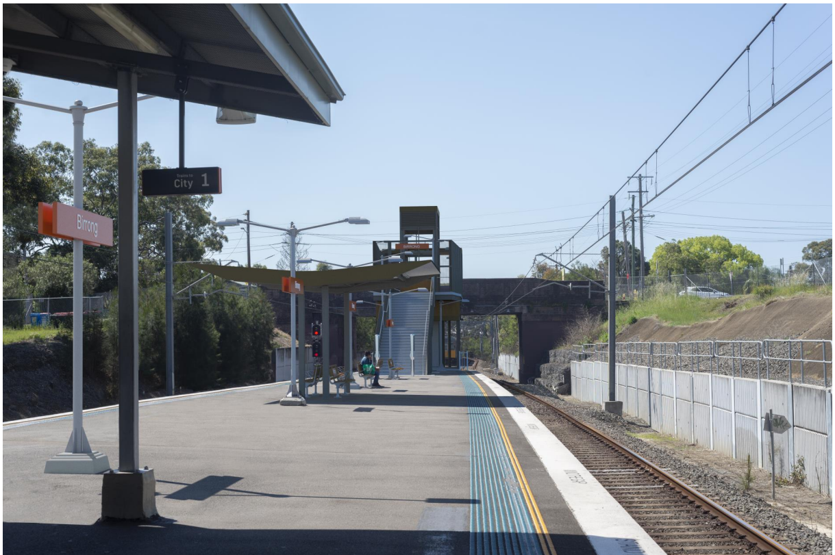
FIGURE 6-3: VIEWPOINT 1 (VP1): SIMULATED IMAGE (PHOTOMONTAGE) OF LIKELY VIEW OF REVISED PROPOSAL FROM STATION 12
