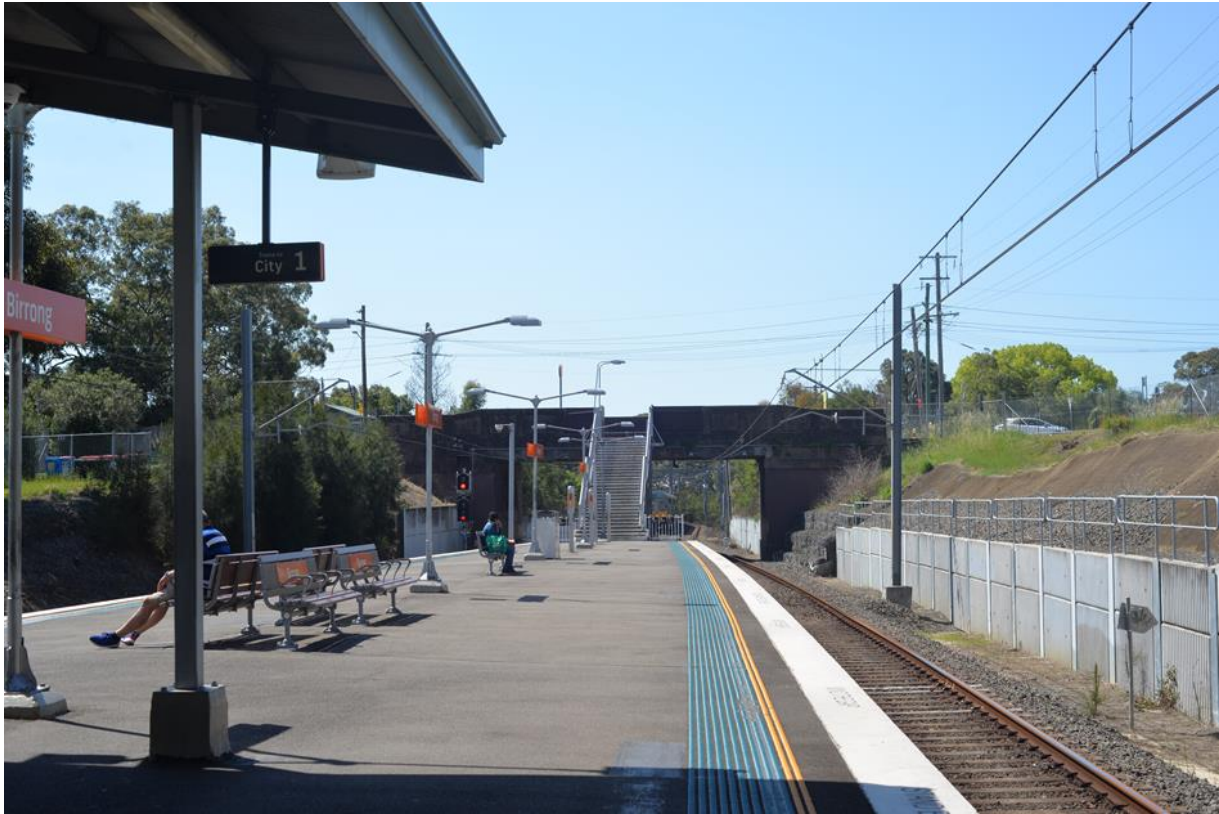
FIGURE 6-2: VIEWPOINT 1 (VP1): EXISTING VIEW FROM EASTERN SIDE OF STATION BUILDING
