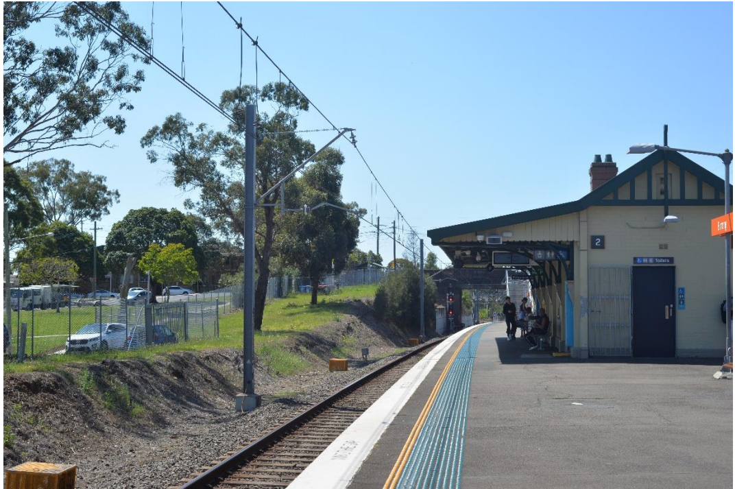
FIGURE 5-2: EXISTING VIEW OF BIRRONG STATION FROM SOUTHERN END OF ISLAND PLATFORM
