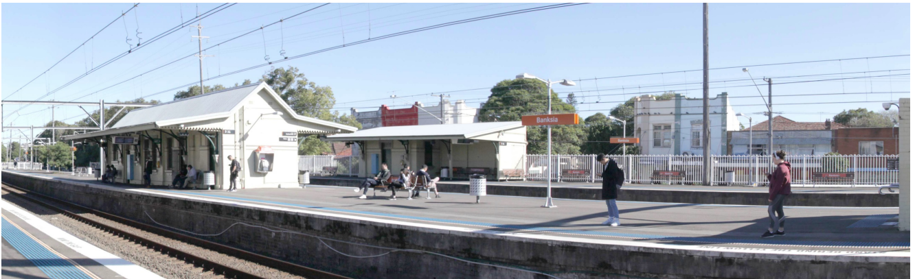
Figure 6.6: Banksia Station Viewpoint 4 – View looking south-west (GPS 56H 328179, 6242374)
