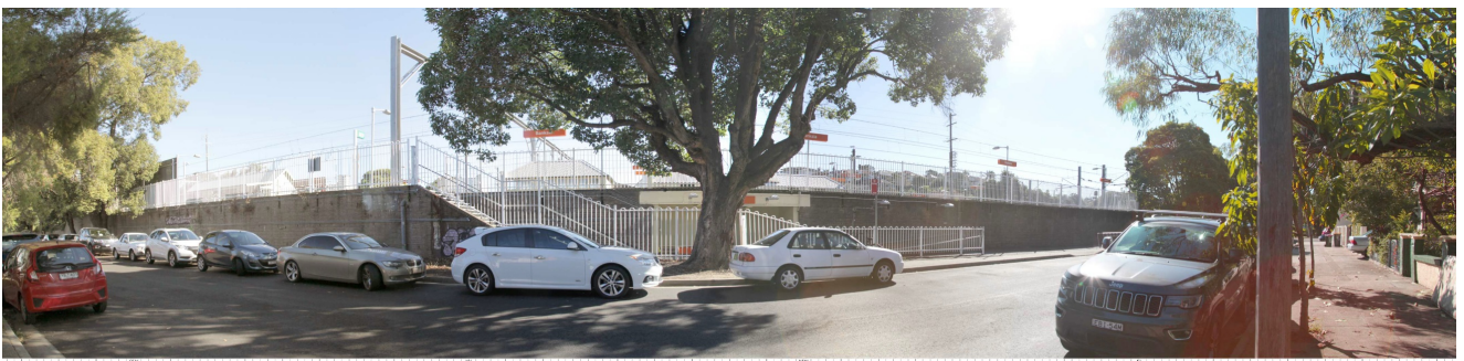
Figure 6.3: Banksia Station Viewpoint 2 – View looking north-west (GPS 56H 328198, 6242378)
