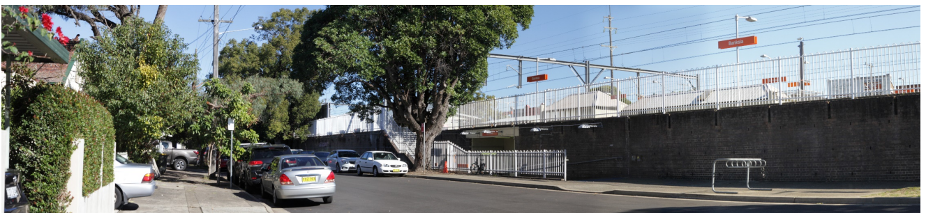
Figure 4.7: Residential interface Hattersley Street – view looking south-west
