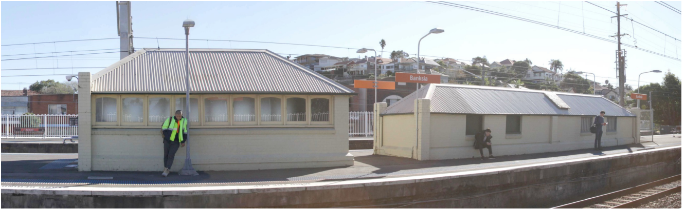
Figure 6.8: Banksia Station Viewpoint 4 – View looking west- north-west
