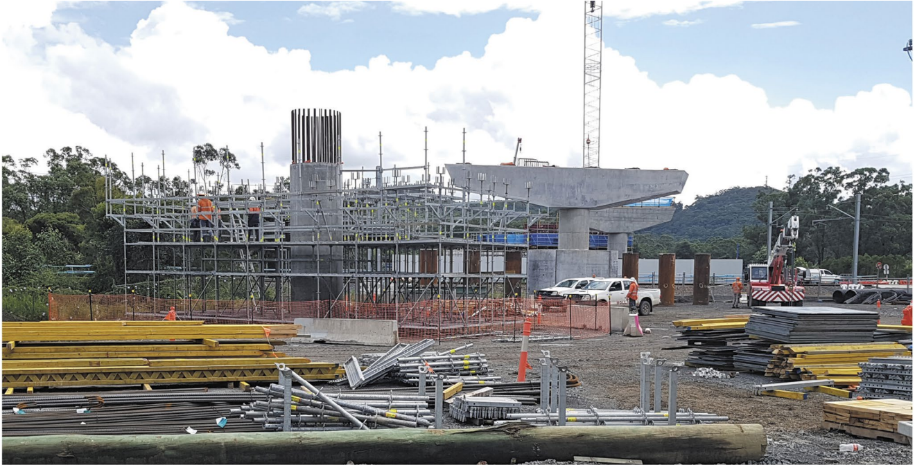
New access bridge under construction
