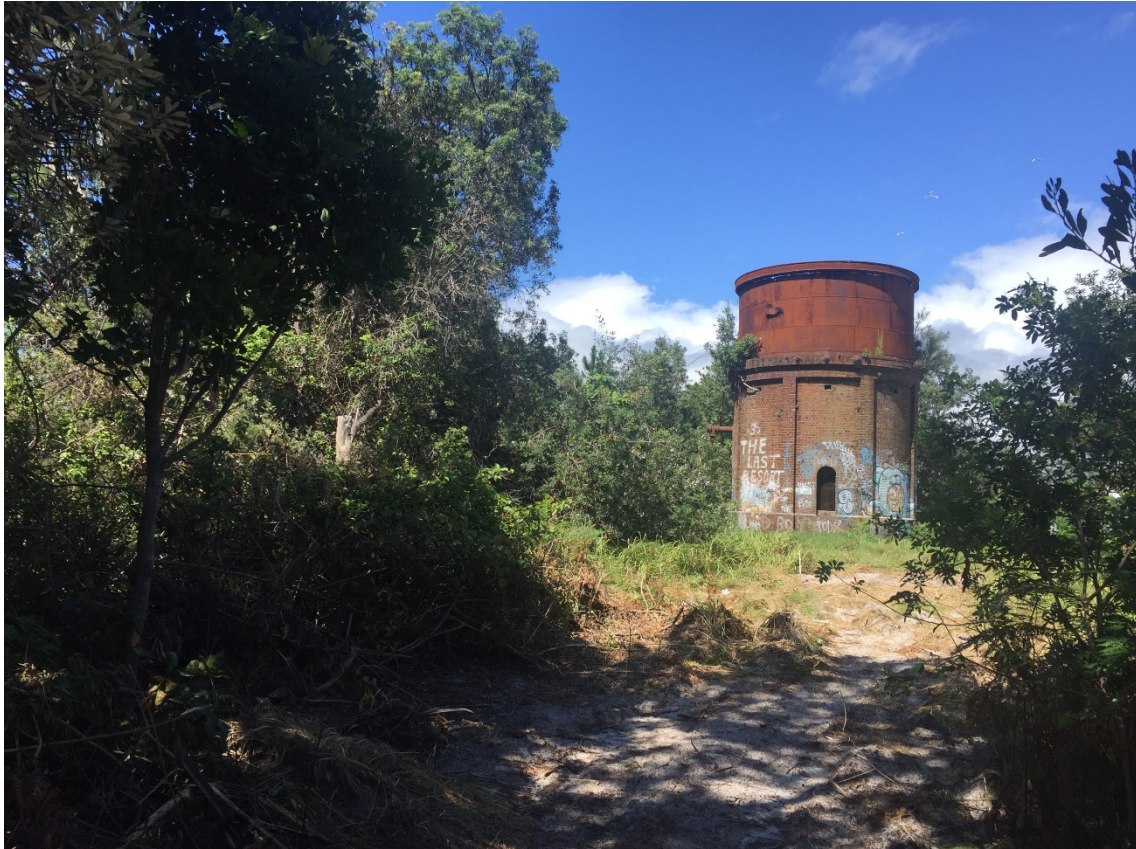
Figure 1-4: Former railway water tower at proposal area (facing south)
