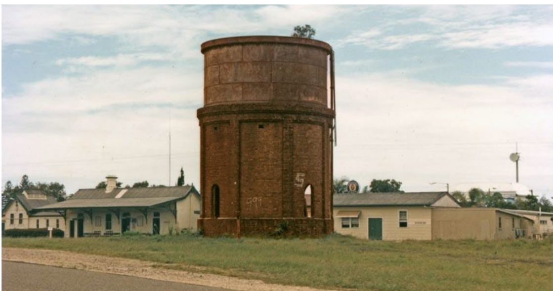
Figure 5-2: Byron Bay Railway Station and water tower in the 1970s (Source: EJ Wright Collection – Richmond Tweed Regional Library)
