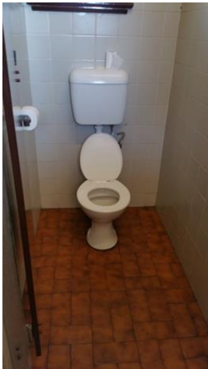
Plate 13 Replacement floor and wall tiles, toilet bowl and cistern in men's toilet
