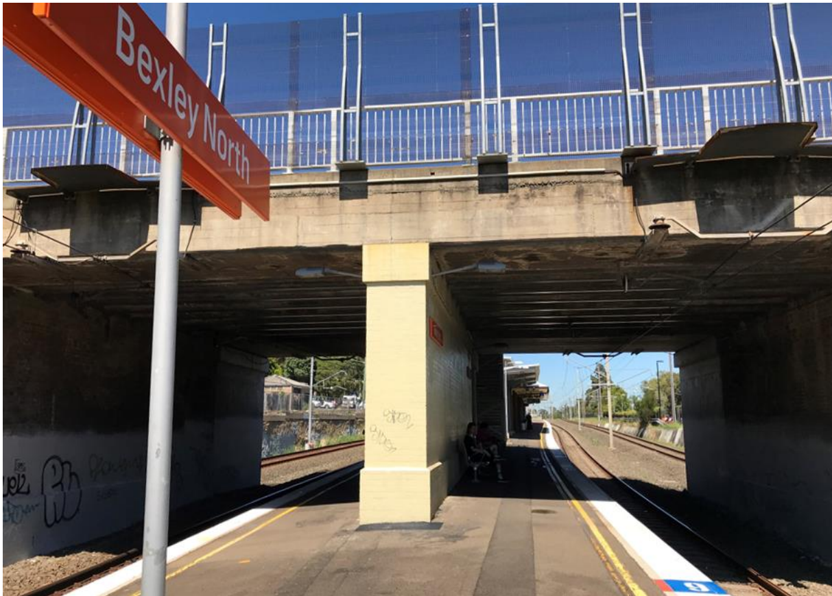
Plate 3 Original brick piers, 2015
