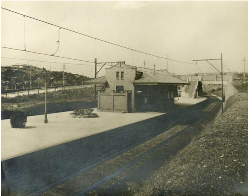
Plate 1 Bexley North Railway Station looking East (Rockdale City Council – Photo file) shows western elevation with screen wall to Male toilets now demolished
