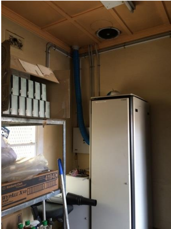
Plate 11 Communications room showing coffered ceiling
