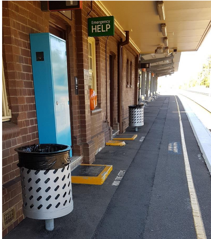
Plate 5 Door and window in southern elevation showing detailing of brickwork around openings
