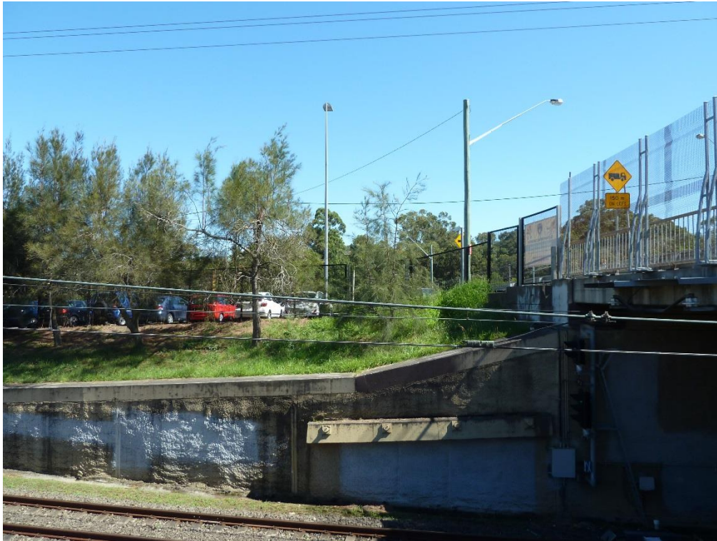
Plate 17 General view of Bexley North Railway Station facing North showing plantings.
