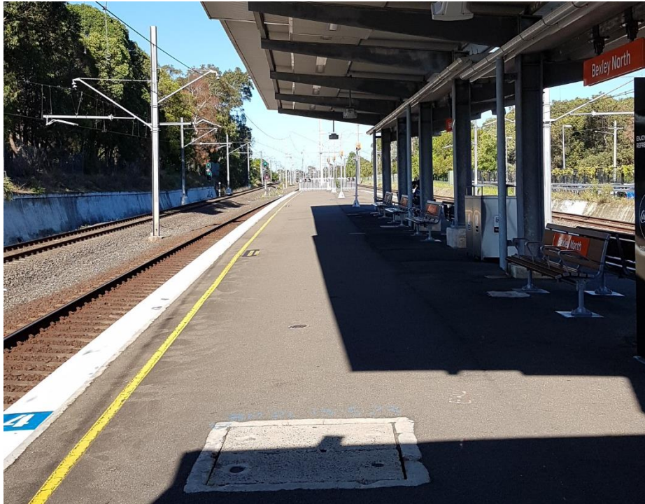
Plate 7 View showing Island Platform. Note weather shelters. View east.
