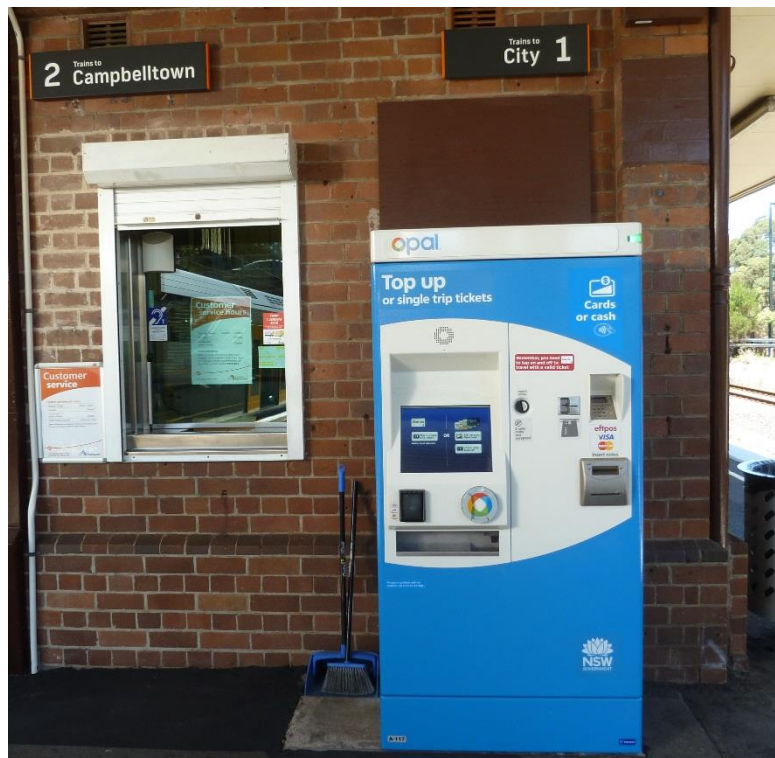
Plate 9 Eastern end of Railway platform building showing modified eastern wall
