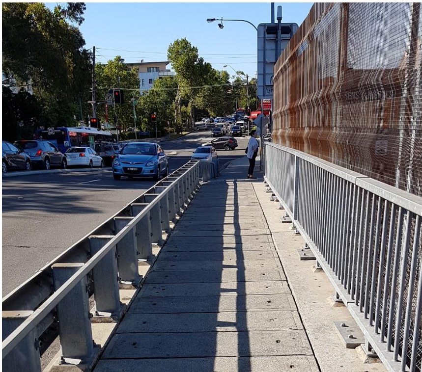
Plate 16 Overbridge pedestrian path.
