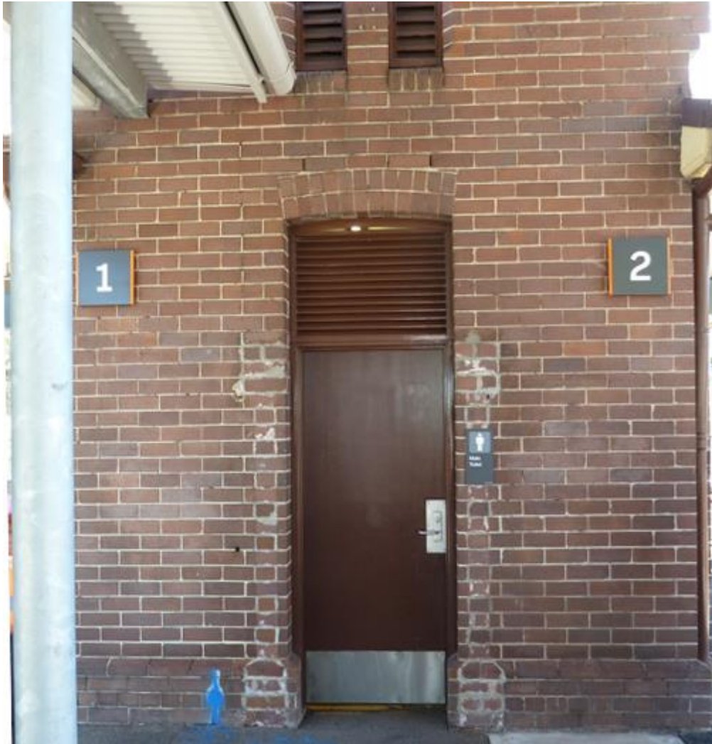
Plate 4 Door in western elevation of platform building showing evidence of screen wall removal.
