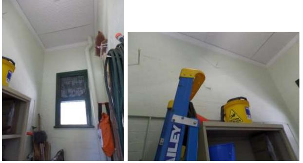
Figure 39. View west (left) and south (right) into the existing Sec/Comms room, showing the small size, the ripple-iron roof and the brick wall proposed for removal.
