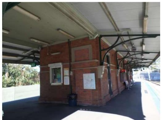
Figure 8. Beecroft - platform building - northern end, showing current ticket window and infilled door opening
