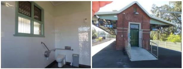
Figure 40. View into existing accessible toilet (left) and the exterior of the accessible toilet, showing the concrete ramp that would be reformed.
