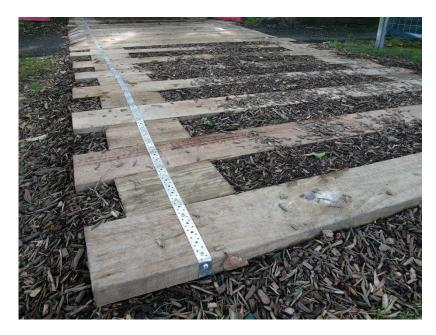
Figure 7 – Showing typical detail for rumble boards.
