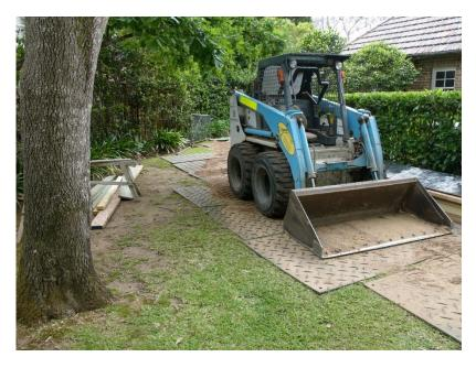
Figure 6 – Showing typical detail for truck mats.
