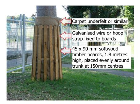
Figure 3 – Detail of Trunk Protection
