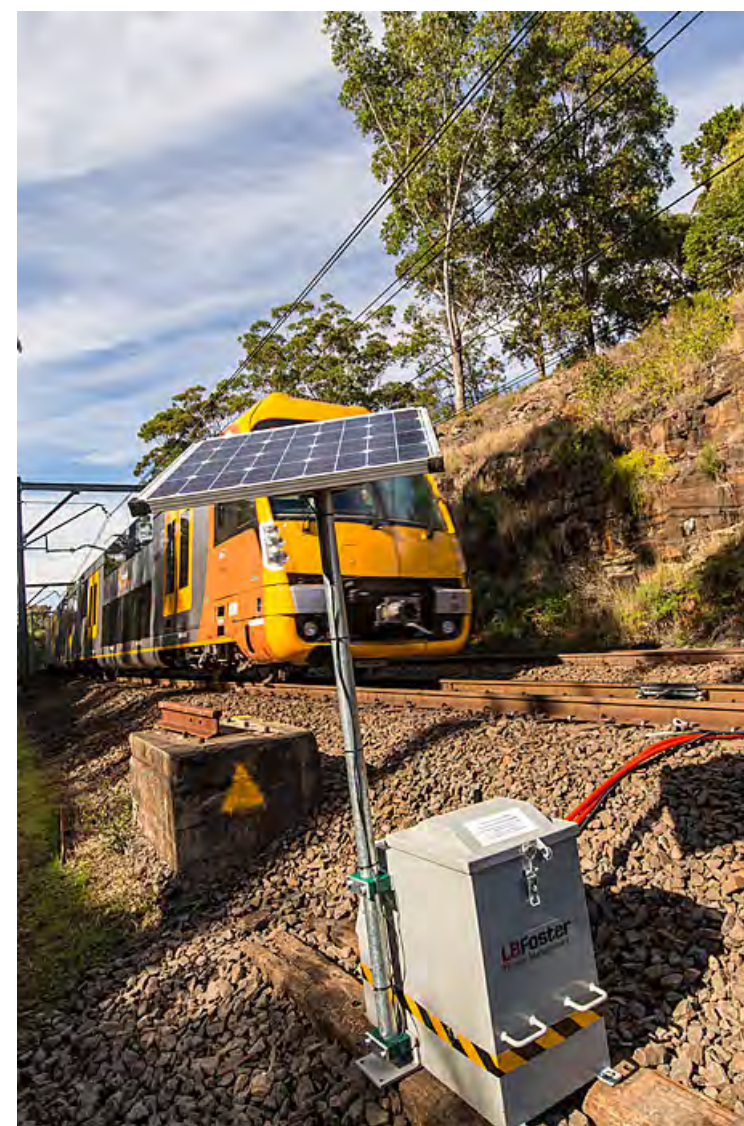
Figure 33 Modern Electronic Lubricators with Remote Monitoring
