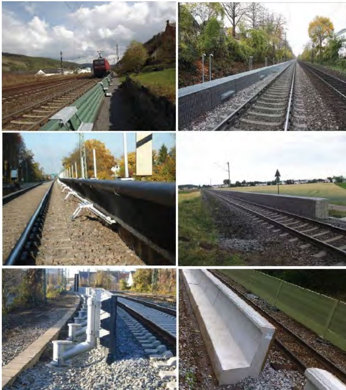
First five barrier example images reproduced from DB Netze Report Innovative Massnahmen zum Lärm- und Erschütterungsschutz am Farhweg Schlussbericht , dated 15 June 2012. Sixth barrier example is a location near Stockholm, Sweden.
