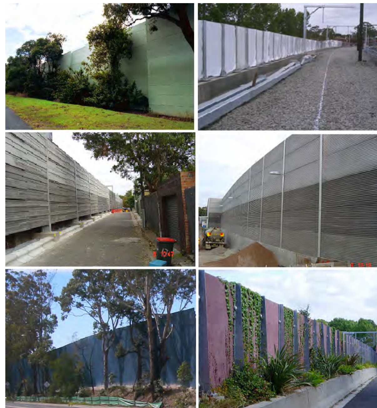
Figure 35 Examples of Conventional Noise Barriers
