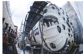
TBM2 is able to lay a concrete slab at Cherrybrook
