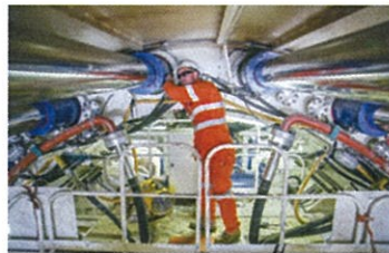
Performing maintenance on a TBM
