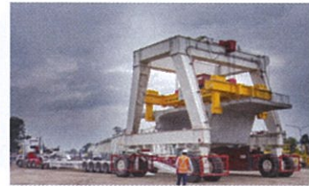
A straddle carrier lifts a 4x12m concrete segment at Kellyville
