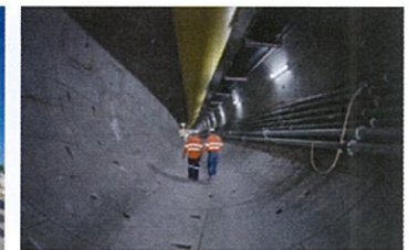
First completed section of tunnel at Bella Vista
