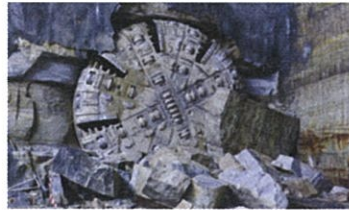
TBM2 Florence breaking through at Showground
