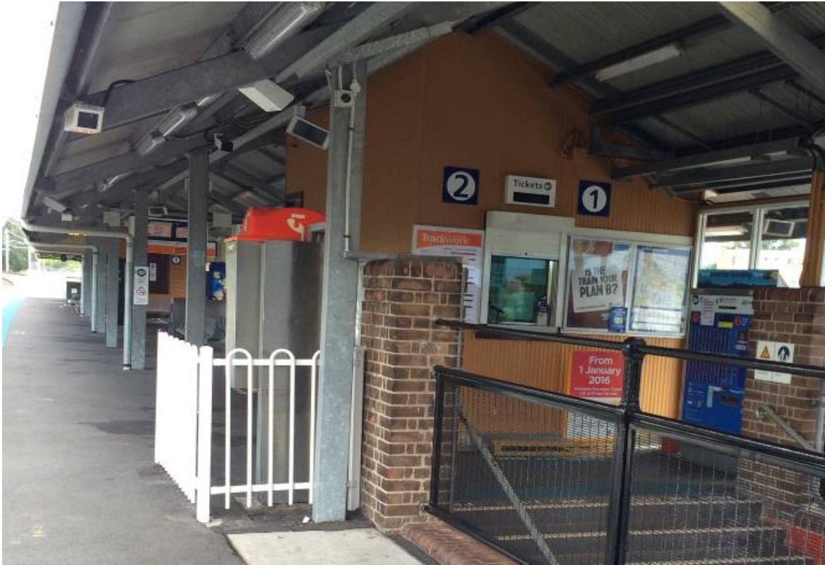
Photo 4 View towards ticket office and top of stairs looking north-west
