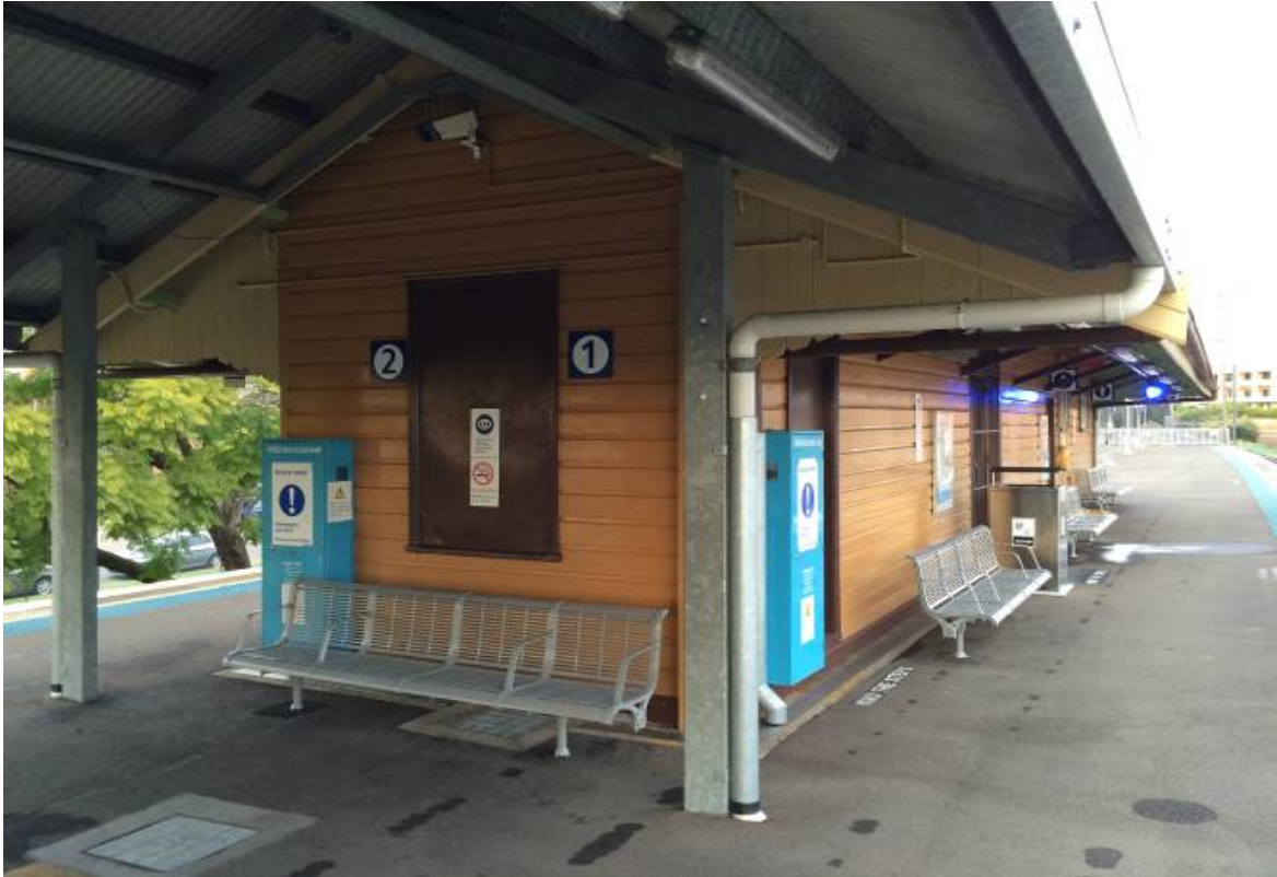
Photo 3 View towards existing platform building looking south-west
