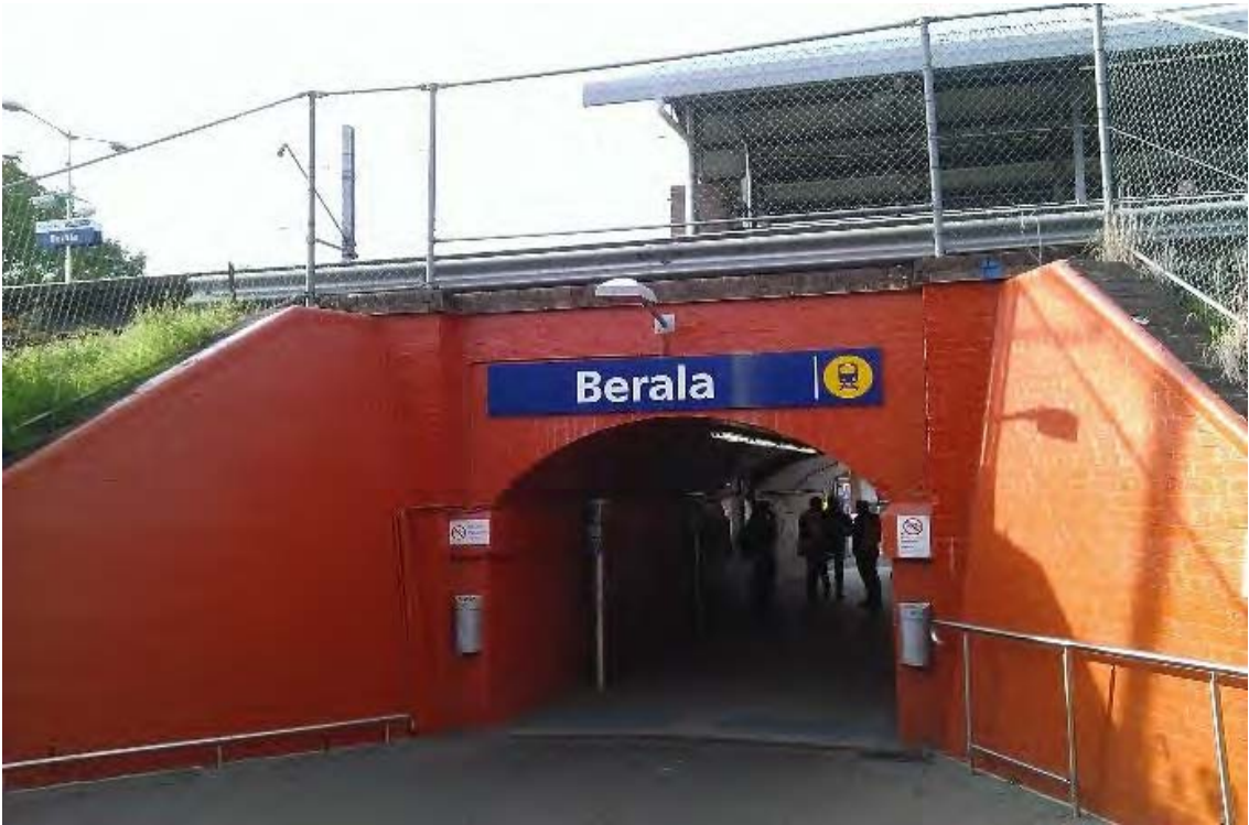
Photo 2 View towards the station from the Woodburn Road underpass entrance
