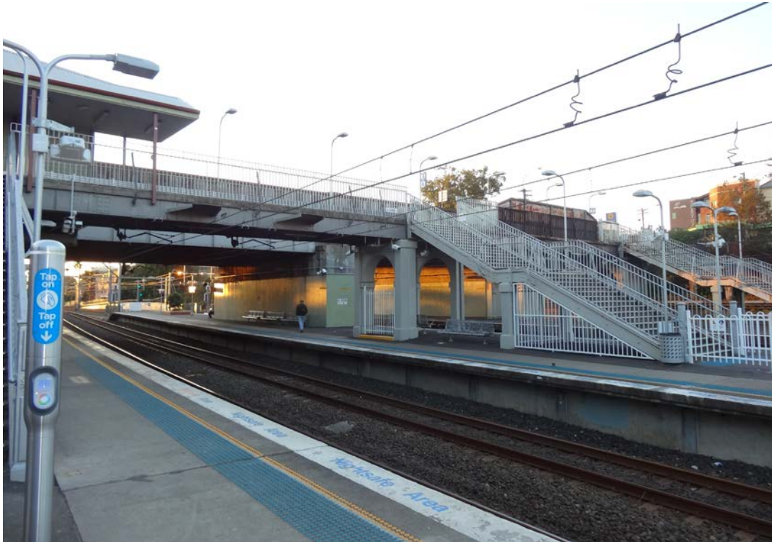
Image 3 View from Platform 5 looking north towards existing footbridge and stairs (to be replaced)
