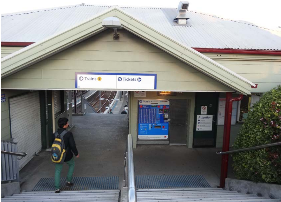
Image 4 View of Meta Street entrance looking south- east down the stairs into the existing booking office (to be replaced with new street-level station entrance)
