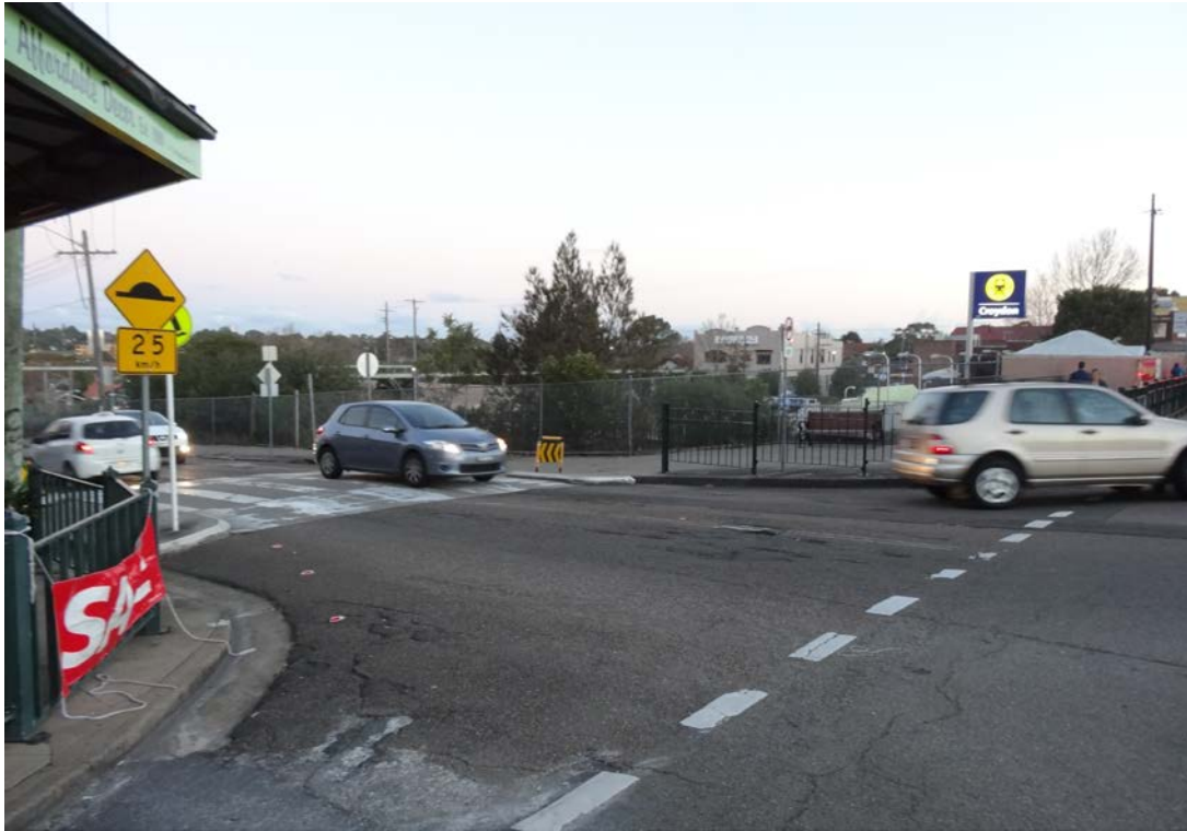
Image 1 View from intersection of Meta Street and Hennessy Street looking south-east towards Croydon Station (note there is no existing direct access to the station from this side)
