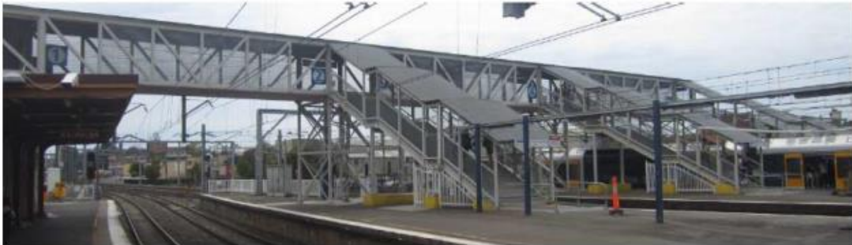
Plate 35 Example of a temporary footbridge used during the Sydenham Station upgrade.
