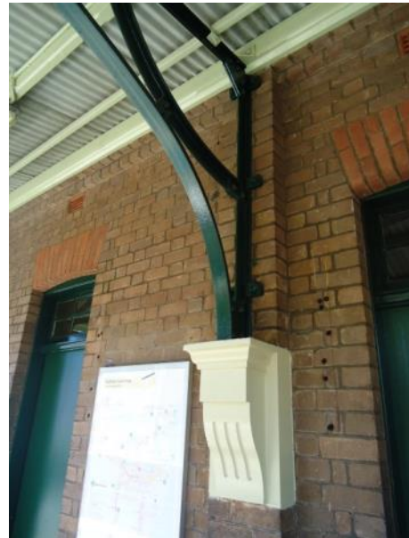
Plate 12 Platform Building 3/4 – detail of concrete corbel and metal bracket for awning.
