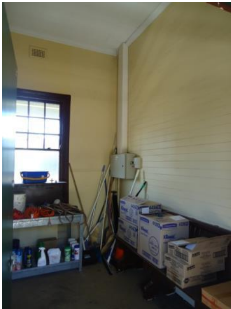
Plate 13 Platform Building 3/4 – interior of store room at northern end of building.
