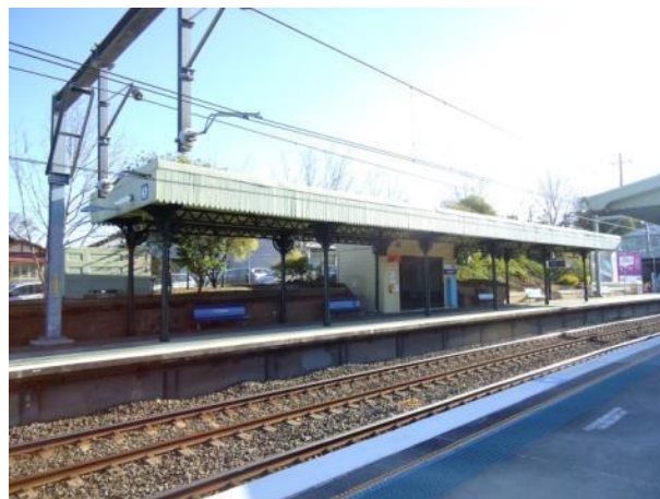
Plate 20 Platform Building 5 – view north west from platform 3/4
