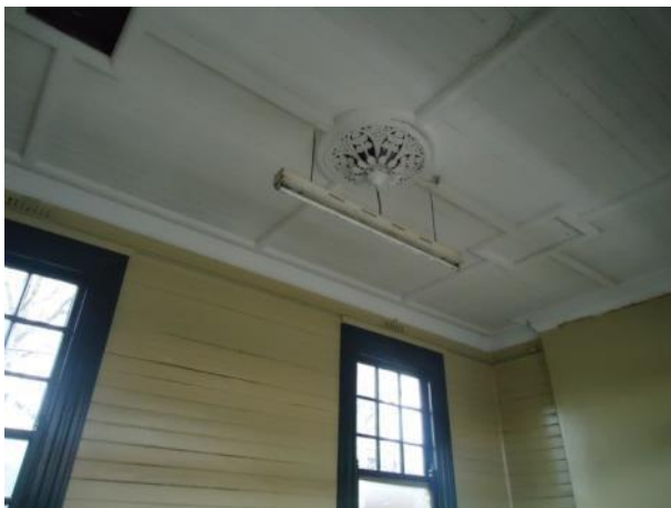
Plate 23 Platform Building 5 – interior showing ceiling detail.
