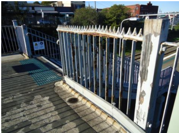
Plate 31 Original balustrade cast iron spiked capping over platform 2 (c.1923).
