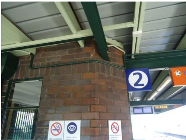
Plate 7 Platform Building 1/2 – attachment of existing canopy, electrical services and wayfinding/information signs.
