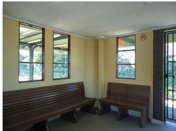
Plate 8 Platform Building 1/2 – interior
