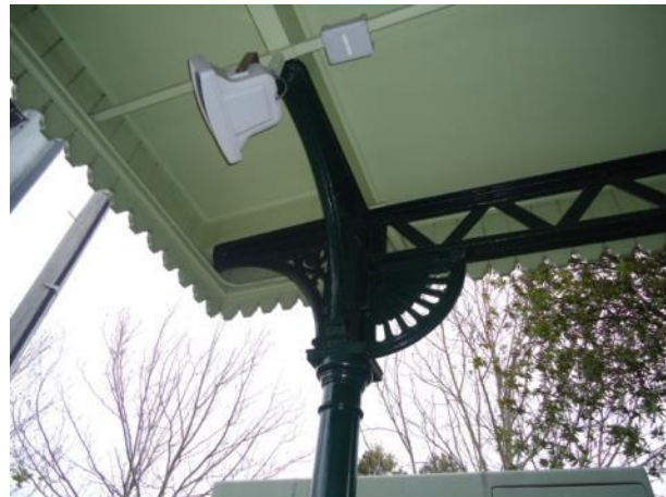
Plate 22 Platform Building 5 – detailing of cast iron work and timber curtain fascia.
