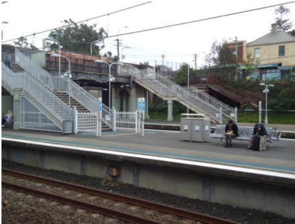
Plate 25 Footbridge showing arrangement of stairs 1, 2 and 3. View north from platform 5.
