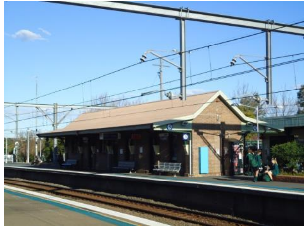
Plate 10 Platform Building 3/4 from platform 2. View south west
