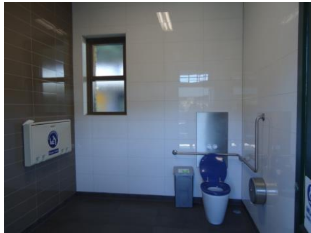
Plate 18 Platform Building 3/4 – interior of recently renovated family accessible/disabled toilet.
