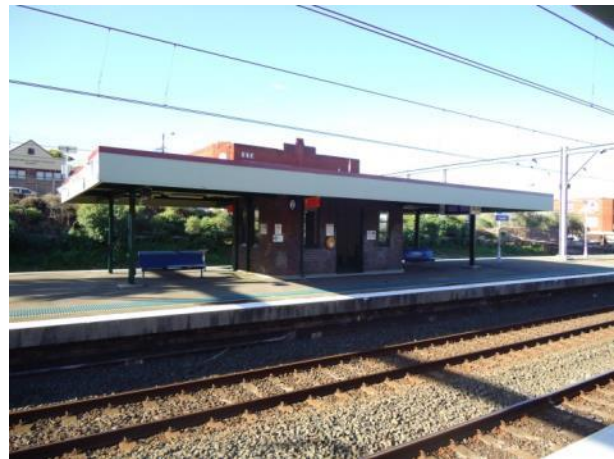
Plate 6 Platform Building 1/2 – view south east from platform 3/4
